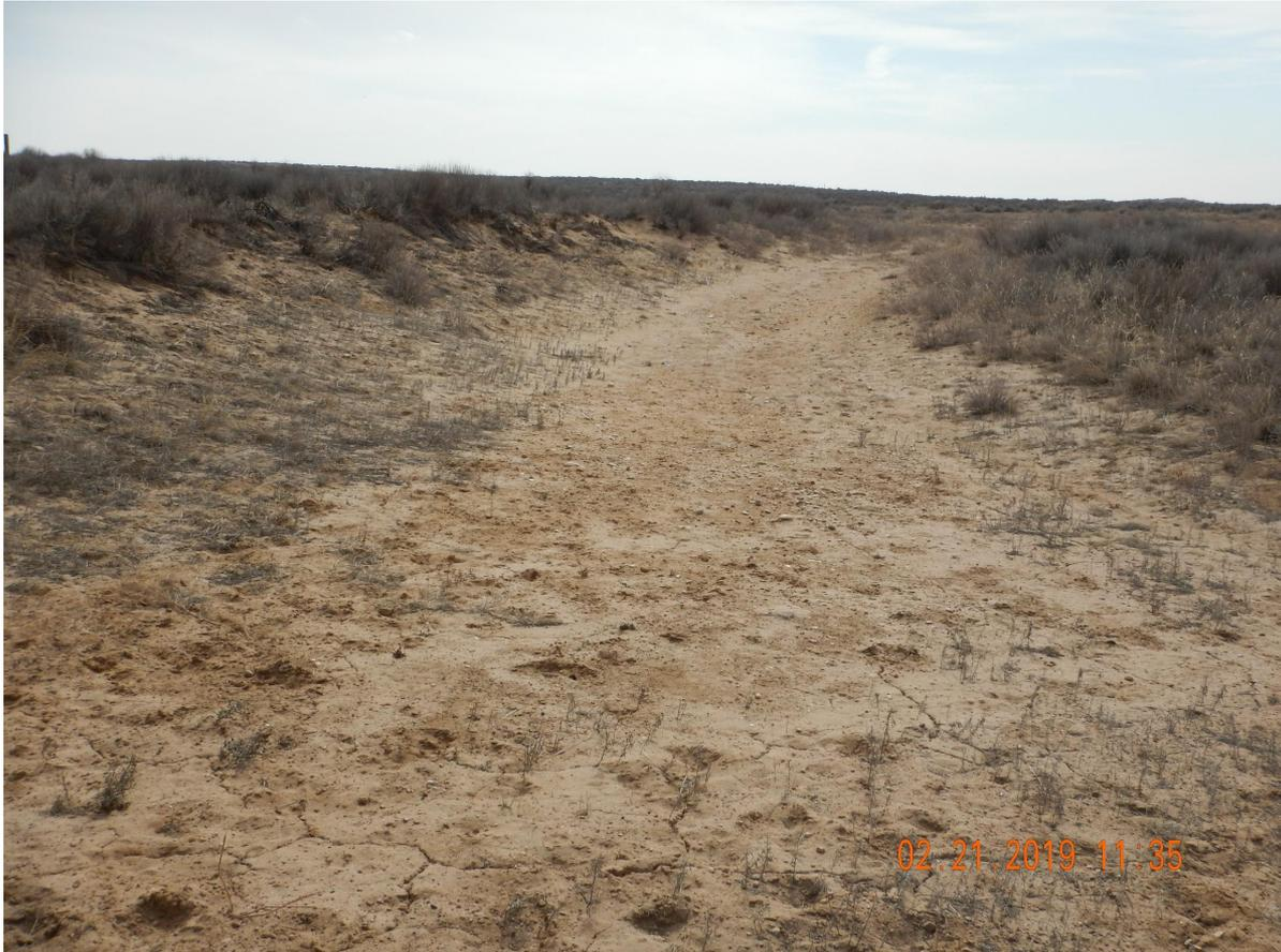
**Photo 1.** Photo taken from the entrance of PA well location access road, facing South. Operator has not performed Final Reclamation activities at the access road. There is no evidence that the access road has been recontoured.
