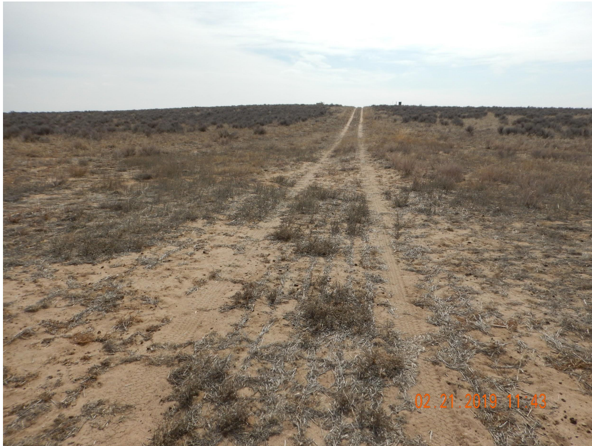
Photo 2. Photo taken from the southern PA well location, facing South. Operator has not performed Final Reclamation activities at the access road. There is no evidence that the access road has been recontoured.
