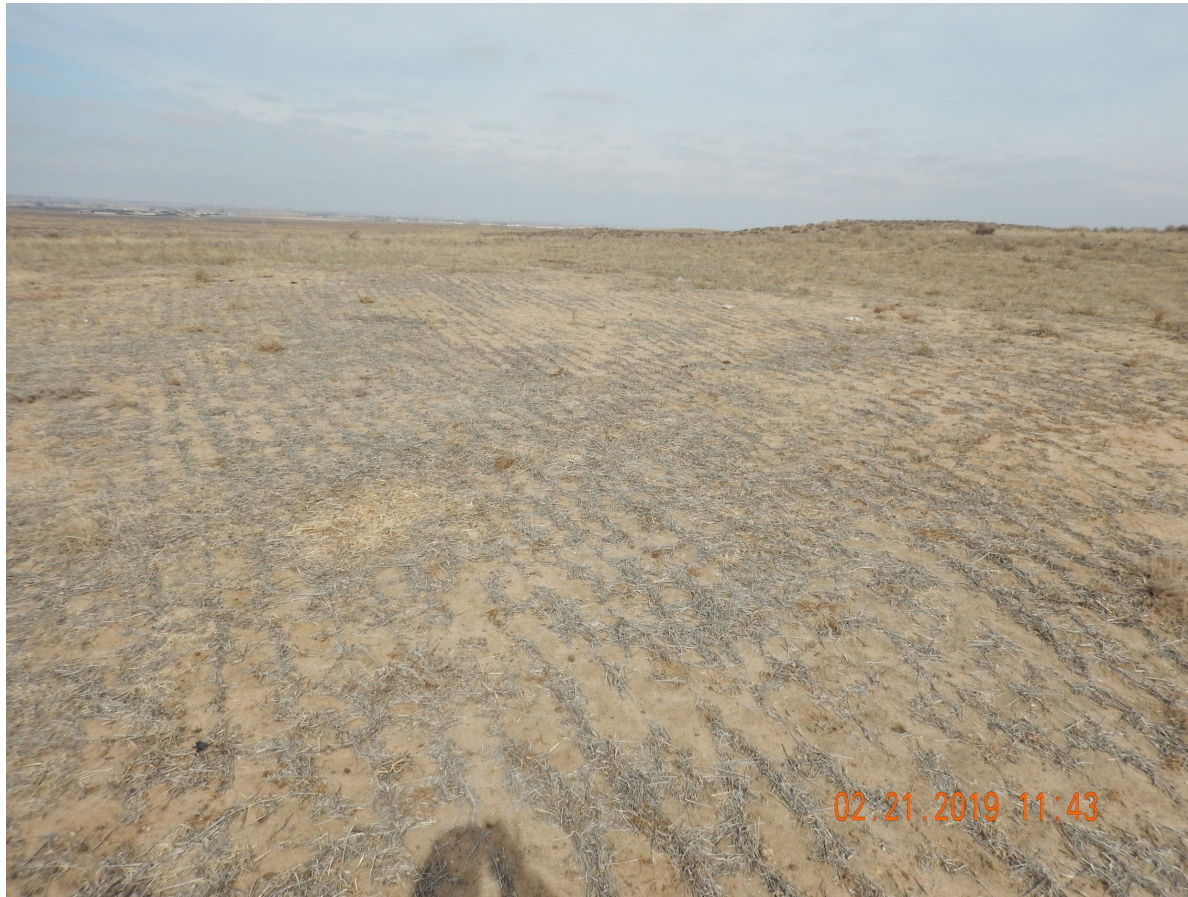
Photo 1. Photo taken from the PA well location, facing North. Appears the Operator has performed Final Reclamation activities at the well location with the evidence of drill rows and mulch. Operator shall continue to monitor and manage this Location until it meets Rule 1004 standards, including weed management.
