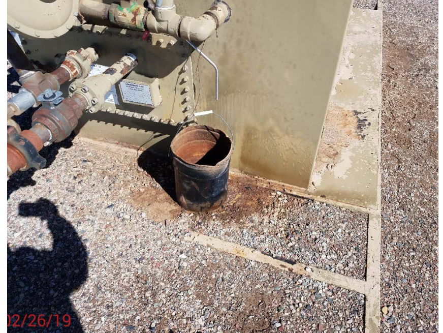
Location Photo #2, Stained ground by separator.
