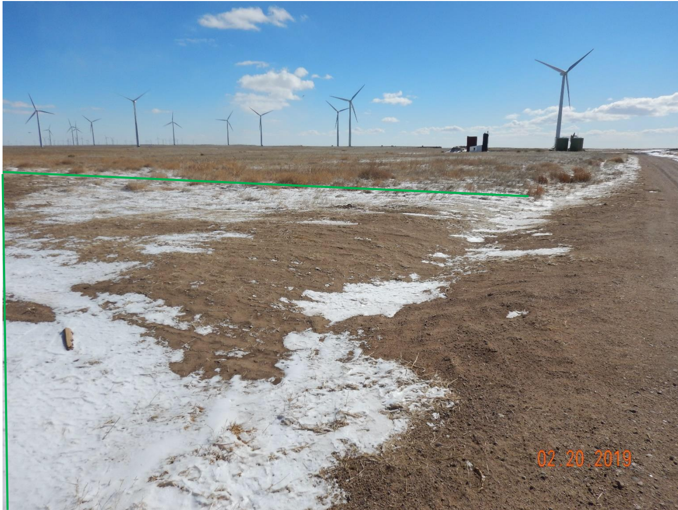
Photo 35: Photo taken from the access road north of the location, facing south towards the location. Photo shows area show areas of disturbance (green) parallel to the access road where operator had removed soil to be brought onto the pad
