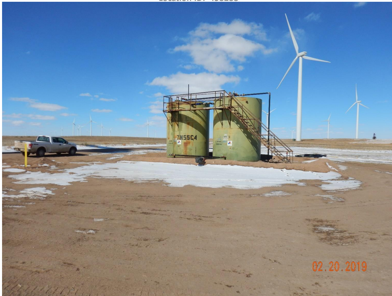
Photo 31: Photo taken from the north end of the location, facing north. Photo shows two (2) 300 bbl AST of “crude oil”. Photo also shows tanks/battery is missing the operator information/signage in accordance with 210.b(2). Berm around battery does not appear to be sufficient in size.
