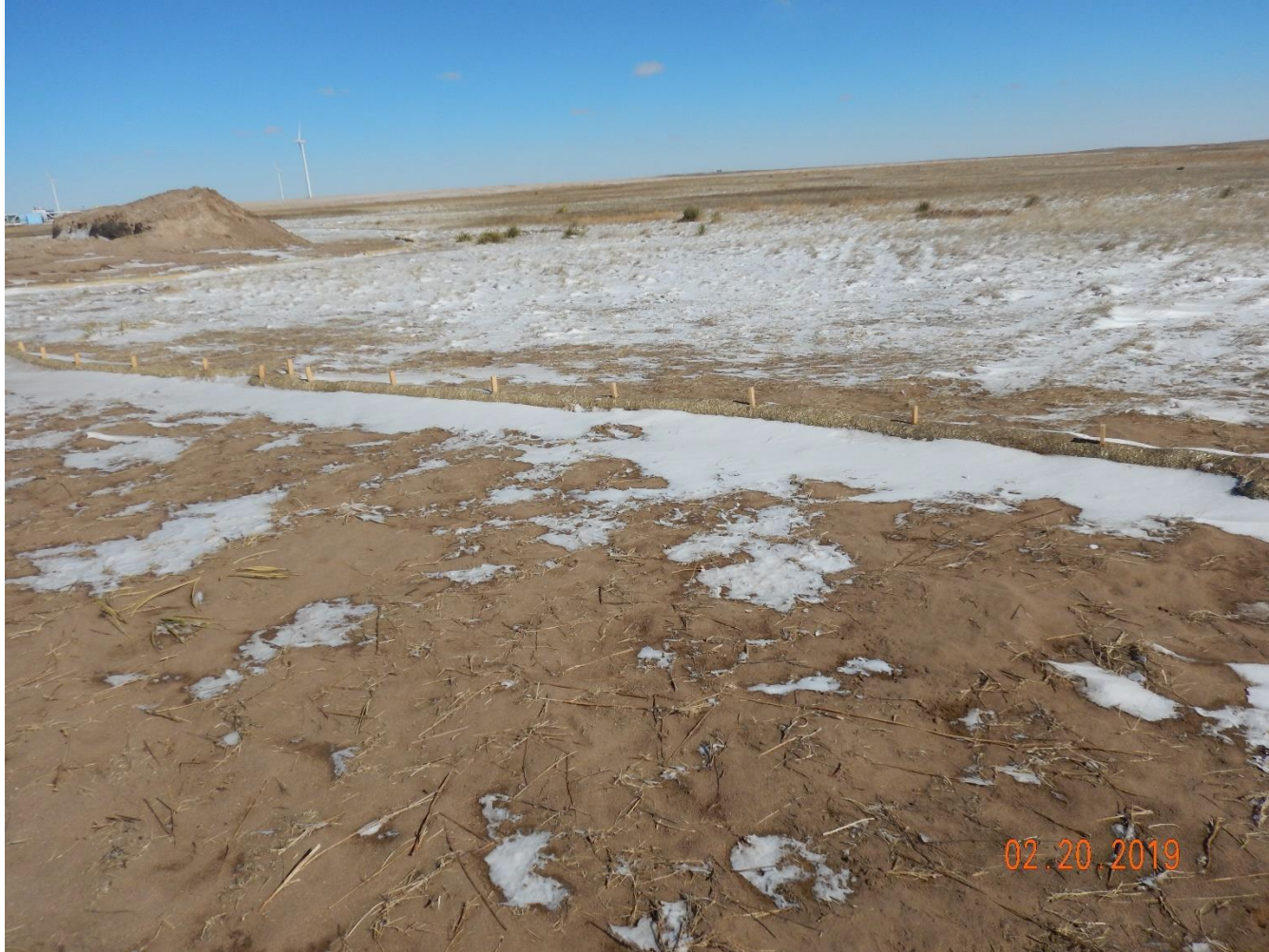
Photo 5: Photo taken from the northeast end of the location, facing east. Photo shows operator has implemented wattles/erosion logs on the eastern, and portions of the northern perimeter of the location. Erosion logs are temporary sediment control barriers and ponding BMPs that intercept sheet flow runoff from disturbed areas, and are required to be trenched and back-filled in order to be in proper functioning condition.
