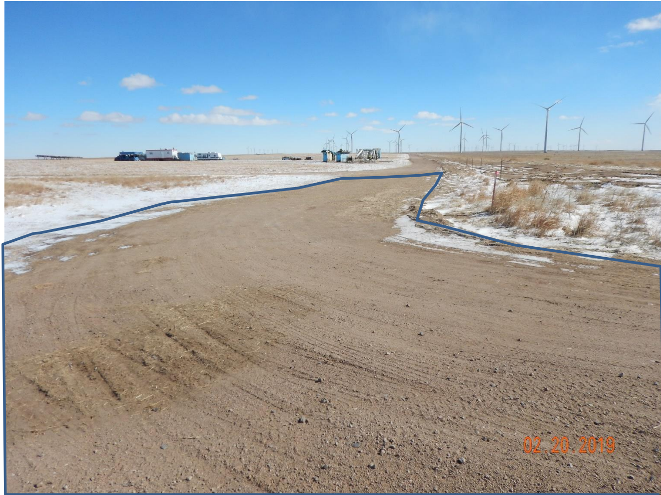
Photo 37: Photo taken from the point where the access road turns from north, to east. Photo shows the only area where operator needed to construct the access road for this location. The road beyond this area had been constructed previously.
