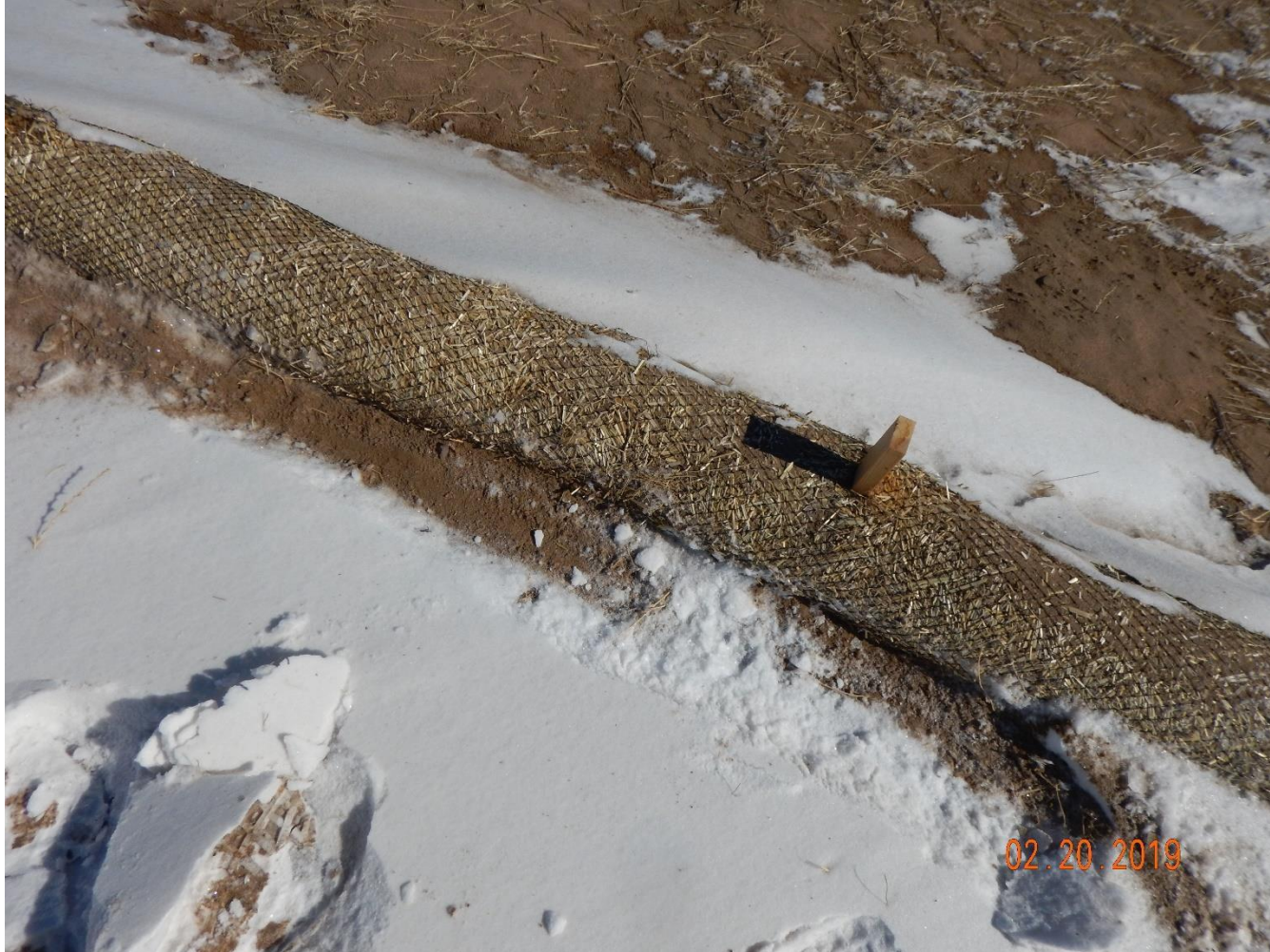
Photo 6: Continued from photo 5. Photo shows Operator only placed/staked the erosion logs upon the surface of the soil; BMPs have not been trenched and back-filled in accordance with good engineering practices and are not in proper functioning condition.
