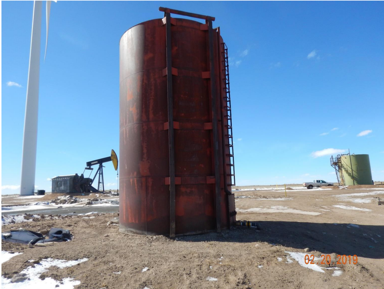
Photo 33: Photo taken from the east end of the location, facing west. Photo shows what appears to be a 300 bbl AST. Tank is missing required signage/labeling in accordance with 210.d. Photo also shows tank is missing required secondary containment in accordance with 906.d(1).
