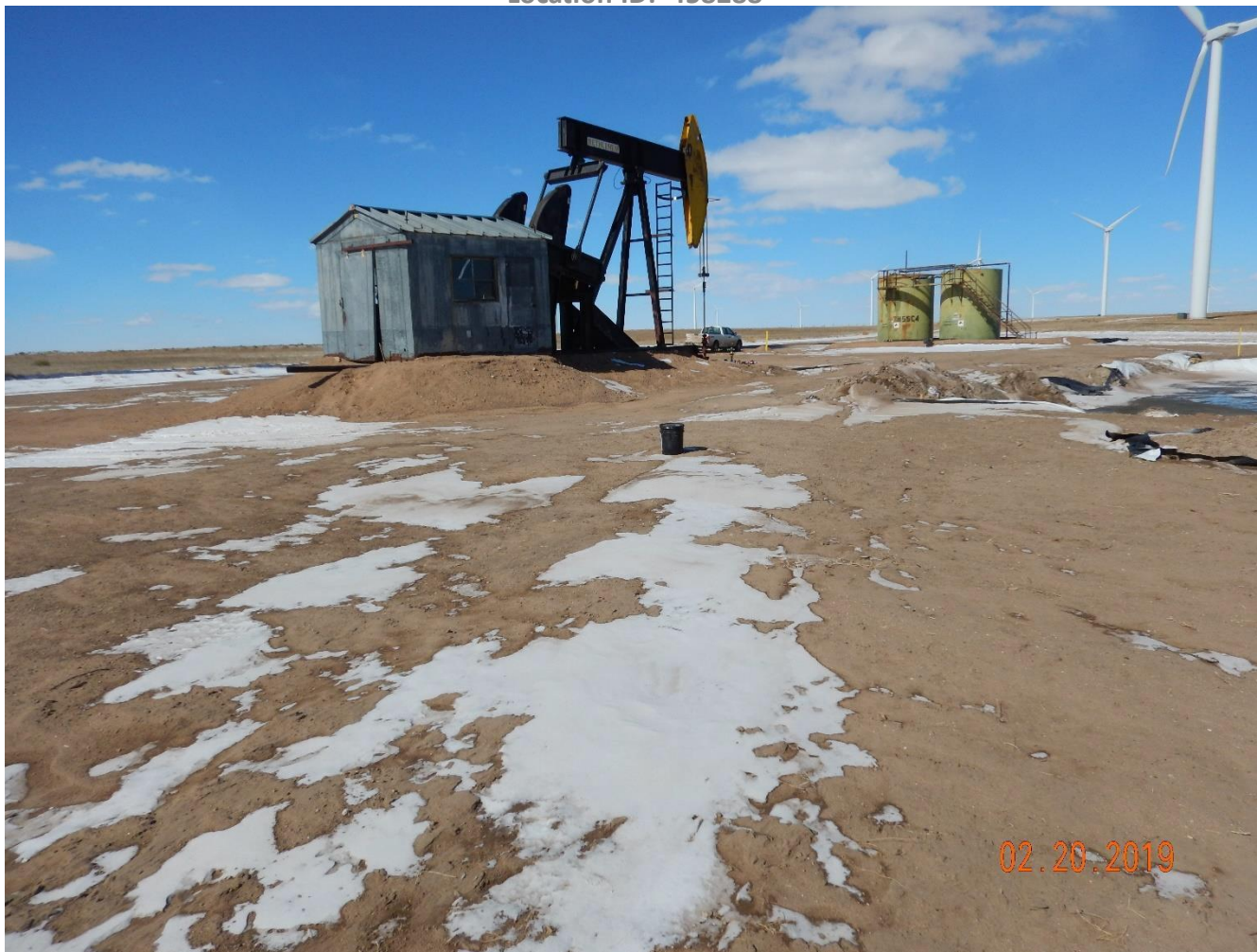
Photo 27: Photo taken from the south end of the location, facing north. Photo shows pumpjack/well and unstabilized soils. Photo also shows a 5 gallon oil bucket being improperly stored on the soil surface of the location.
