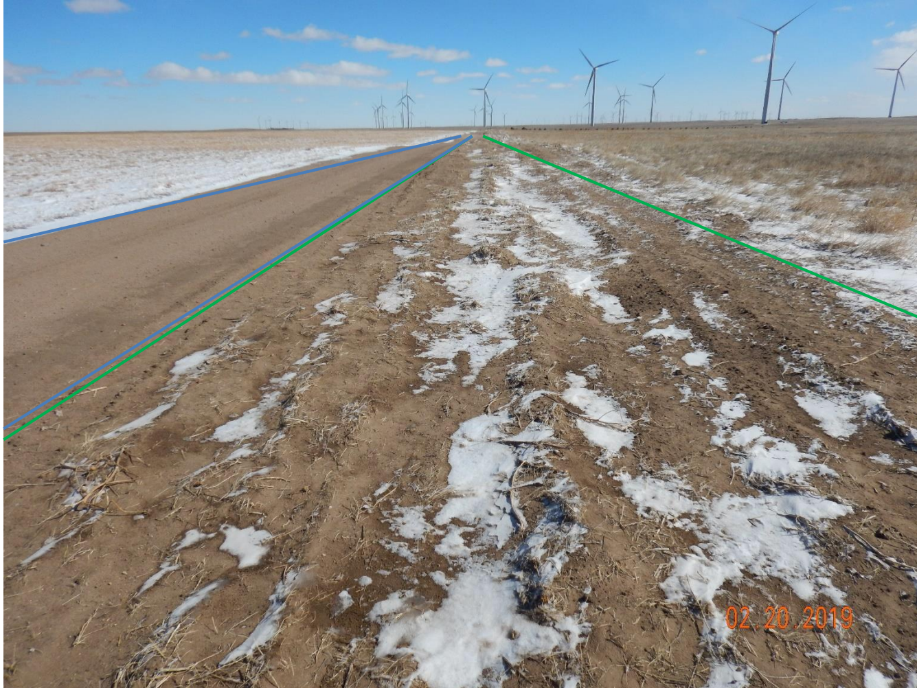
Photo 41: Photo taken from the access road north of the location, facing east. Photo shows areas of disturbance (green) parallel to the access road (blue) where operator had removed soil to be brought onto the pad
