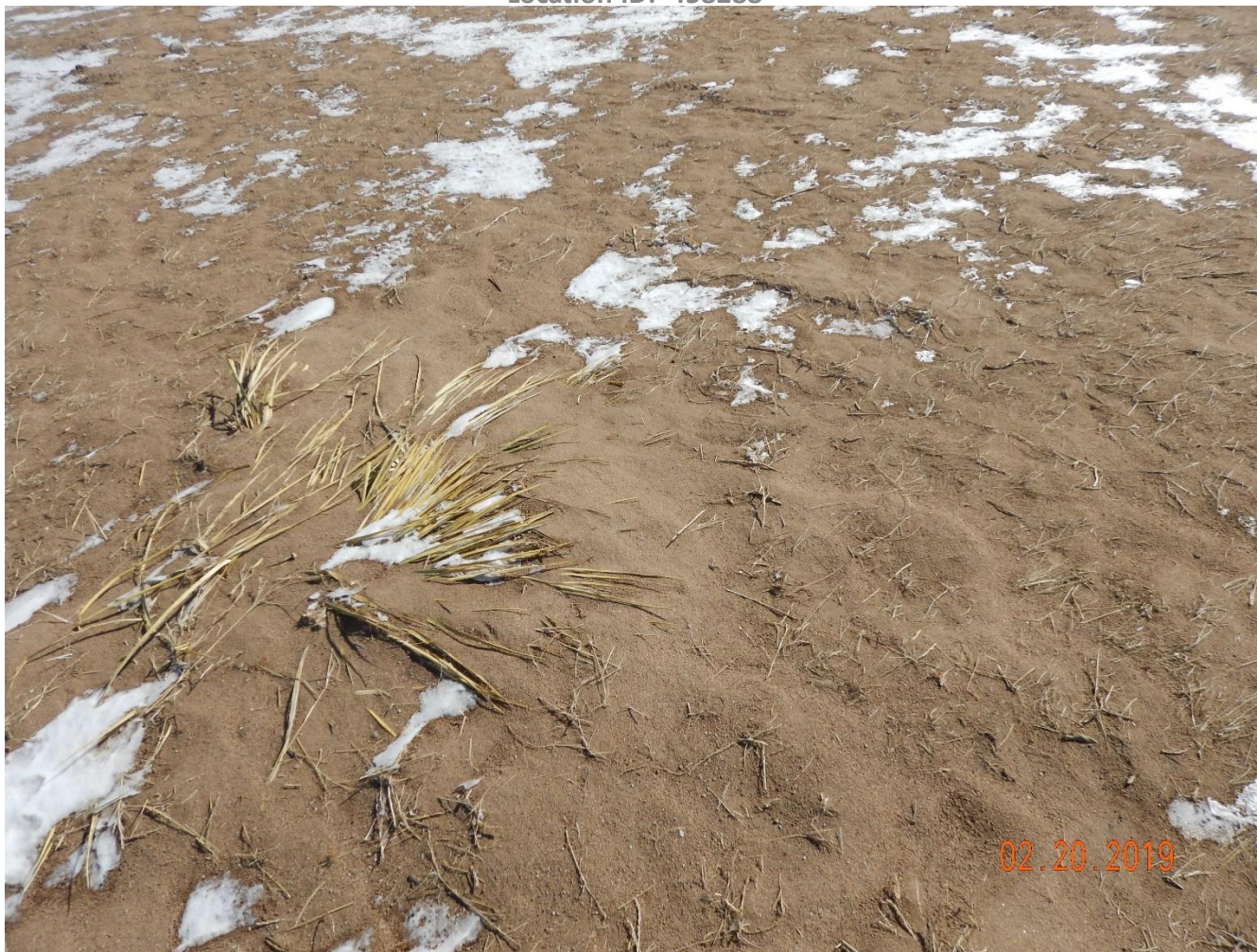
Photo 4: Photo taken from the south end of the location. Photo shows area where operator had brought soil to “build up” the pad. Operator previously stated that “~3 feet of soil will be placed on the location to build up the pad”. Photo shows vegetation (yucca, grass) is visible within the material brought on location suggestion either 1) Operator failed to stabilize the soils brought onto the pad and wind erosion has removed the material, or 2) Operator failed to import a sufficient amount of material to build to pad and protect the topsoil below. Regardless, operator has failed to take appropriate measures to protect the topsoil and the natural features.
