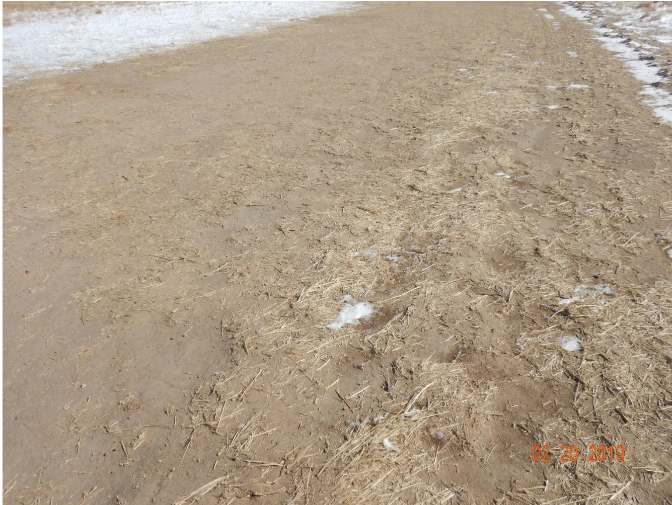
Photo 38: Continued from photo 37. Photo shows vegetation on the area of the new section of access road. Operator does not appear to have constructed the road (salvaged topsoil, imported road base) but rather traveled over the surface until a road was created. This is not protective of topsoil.
