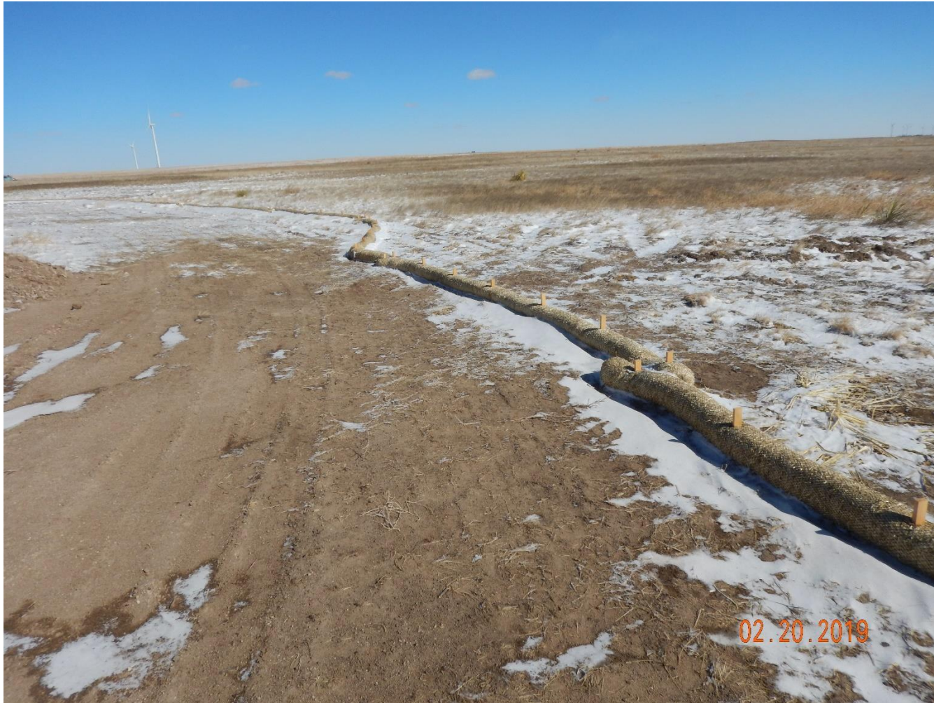
Photo 7: Continued from photo 5. Photo shows Operator improperly installed erosion logs. See comments under photo 6.
