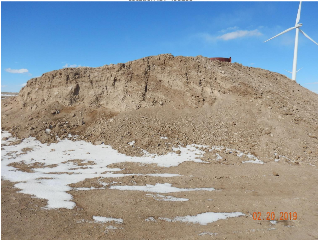
Photo 9: Photo taken from the south end of the pit soil stockpile, facing north. The previous inspection documented that the topsoil and subsoil horizons from the pit was not separated and stored in accordance with 1002.b. This photo continues that documentation. Additionally, rule 1002.c requires that "All stockpiled soils shall be protected from degradation due to contamination, compaction and, to the extent practicable, from wind and water erosion during drilling and production operations". Photo shows soil stockpile remains loose, unstabilized material at risk to wind and water erosion. Operator has failed to sufficiently stabilize the soil stockpile in accordance with 1002.c
