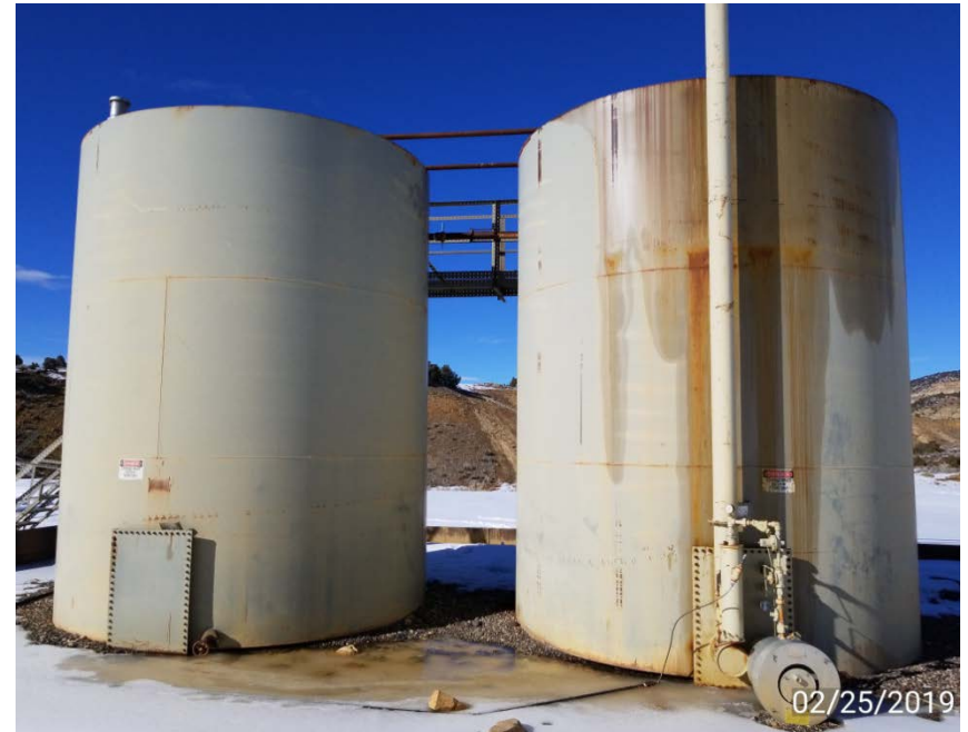
Photo 4. Tank battery looking north. Oil staining on side of oil tank.
