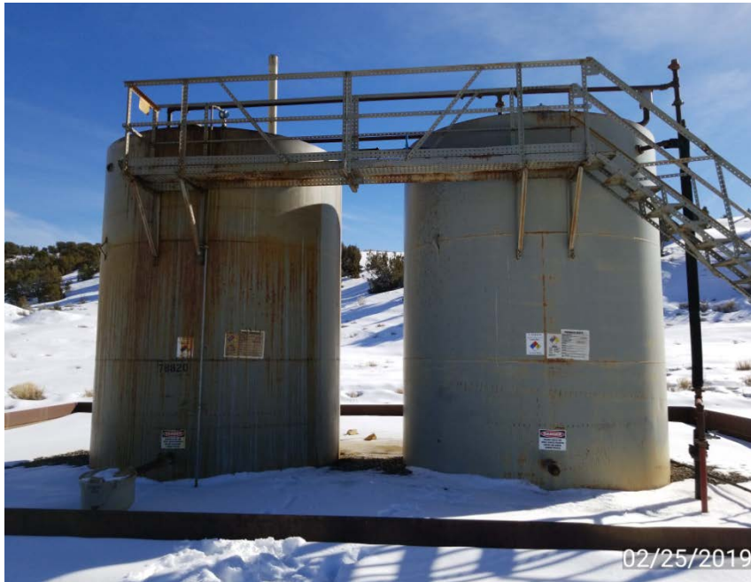
Photo 3. Tank battery looking south. Oil staining on side of oil tank.
