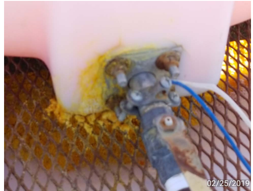
Photo 6. Xylene / ethylbenzene container leaking into secondary containment.
