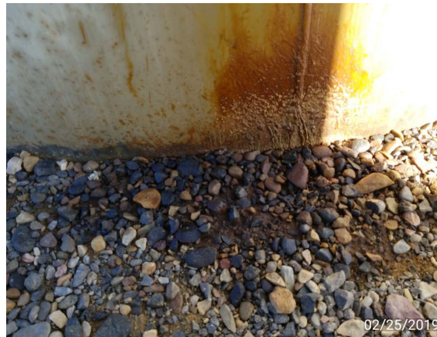
Photo 2. Oily waste at base of crude oil tank.
