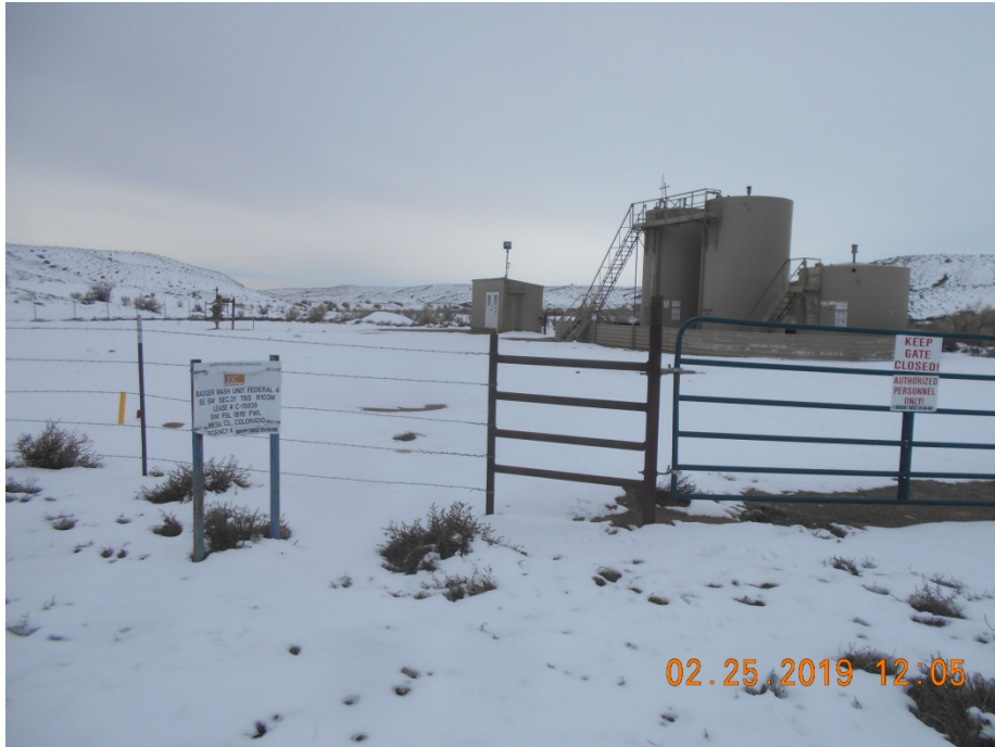
Overview of location looking SW.
