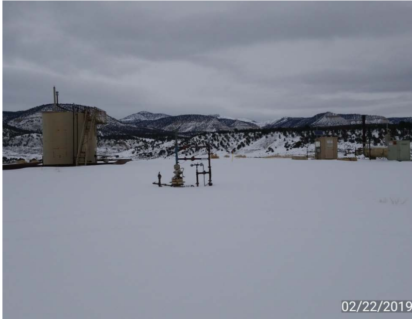
Photo 1. Location looking west.
