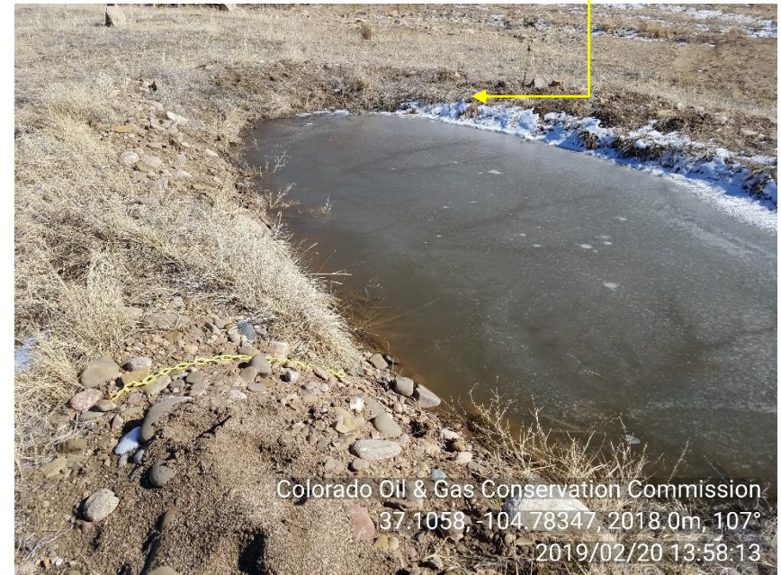
PHOTO 4: PRODUCED WATER LEVEL IN PIT APPEARS TO BE VERY CLOSE TO FREEBOARD/ FREEBOARD MARKER NOT INSTALLED CORRECTLY
