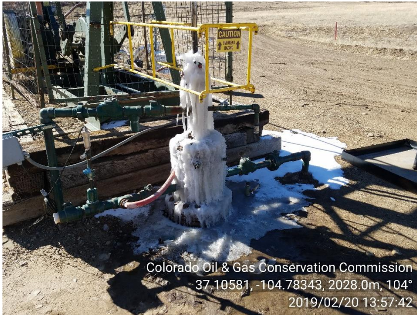
PHOTO 3: ICE BUILDUP ON WELLHEAD APPEARS TO BE PRODUCED WATER FROM LEAKING ROD PACKING
