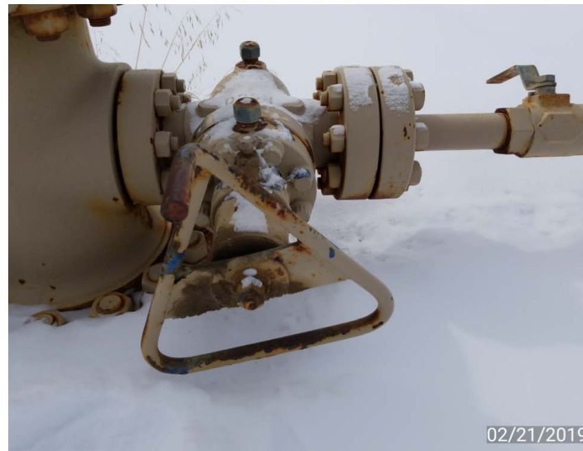
Photo 2. Casing well head valve leaking gas.
