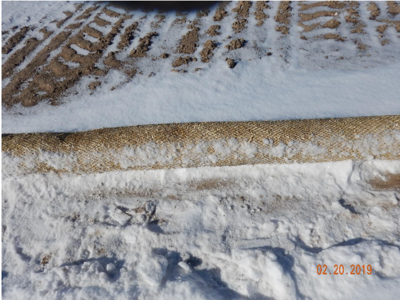
Photo 14: Continued from photo 13. Photo shows erosion log has not been trenched and backfilled in accordance with good engineering practices
