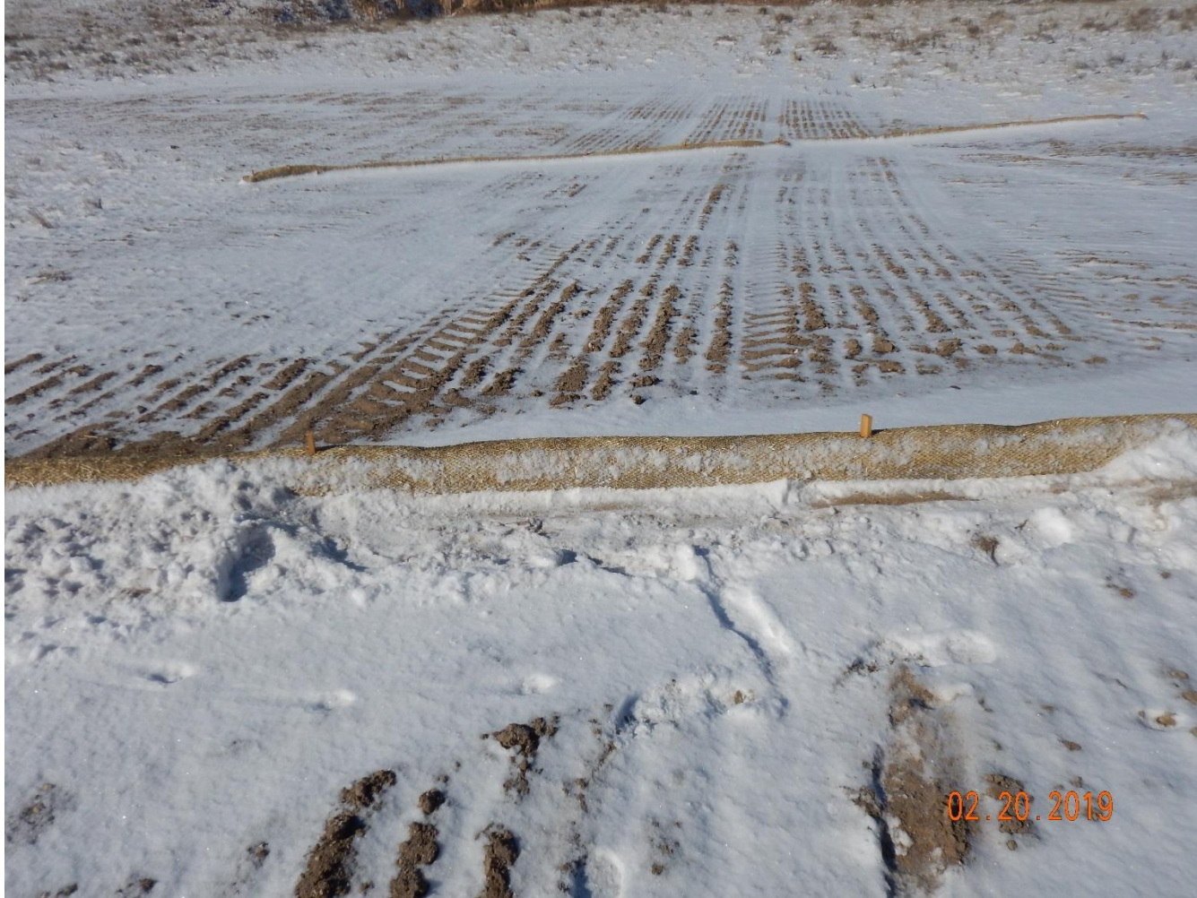
Photo 13: Photo taken from the southwest interim areas (southwest of pit) facing west. Photo shows erosion log has not been trenched and backfilled in accordance with good engineering practices. See comments under photo 2.
