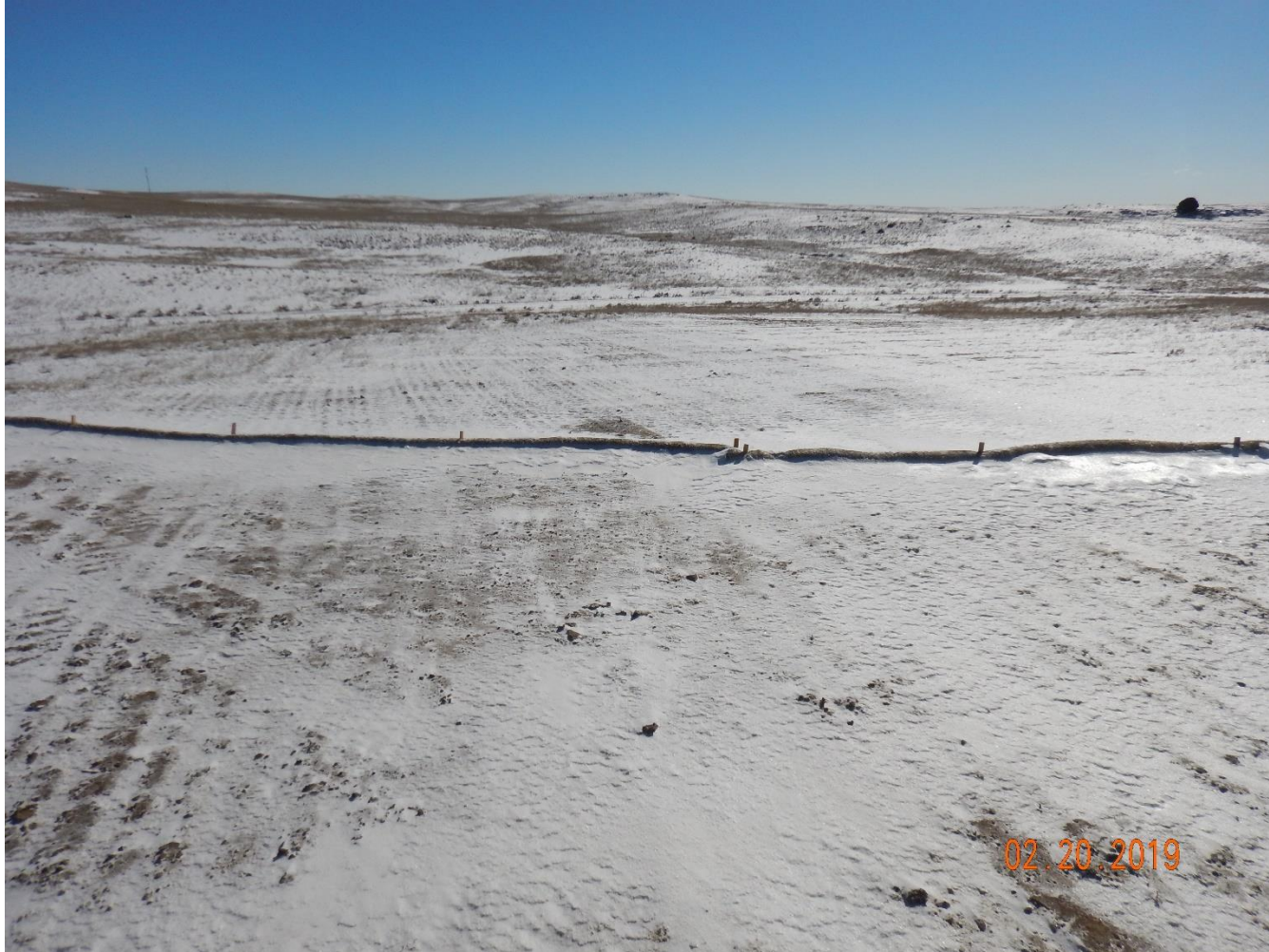
Photo 7: Photo taken from the southeast interim areas (Southeast end of pit), facing southeast. Photo of erosion log. See comments under photo 2.
