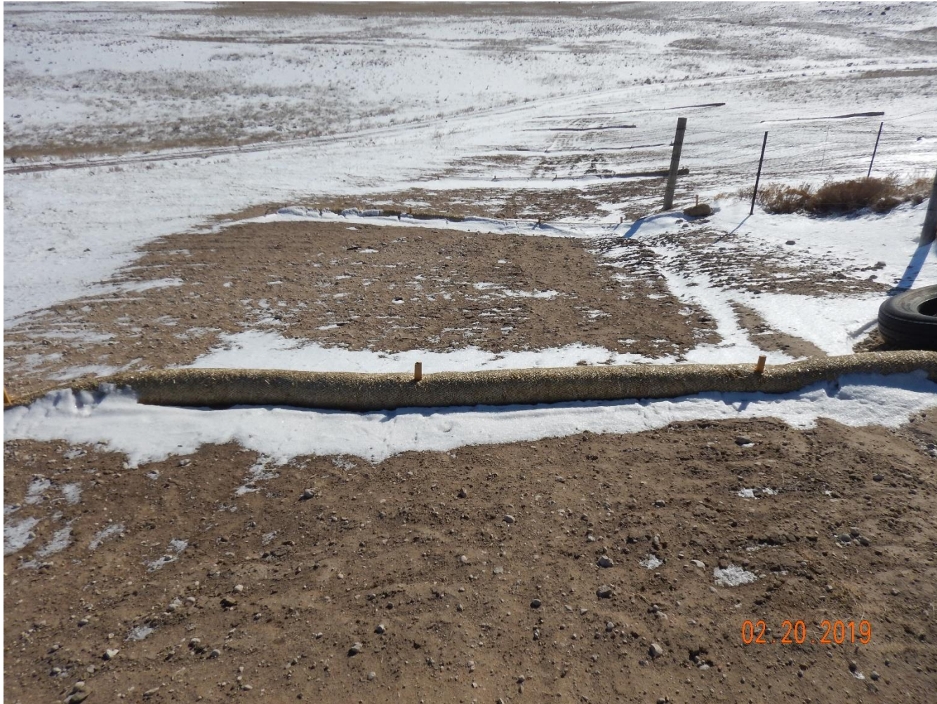
Photo 2: Continued from photo 1. Photo shows erosion log BMP. Erosion logs are sediment control barriers and ponding BMPs that intercept sheet flow runoff from disturbed areas, and are required to be trenched and back-filled in order to be in proper functioning condition. Photo shows Operator appears to have only placed/staked the erosion logs upon the surface of the soil; BMPs have not been trenched and back-filled in accordance with good engineering practices and are not in proper functioning condition.
