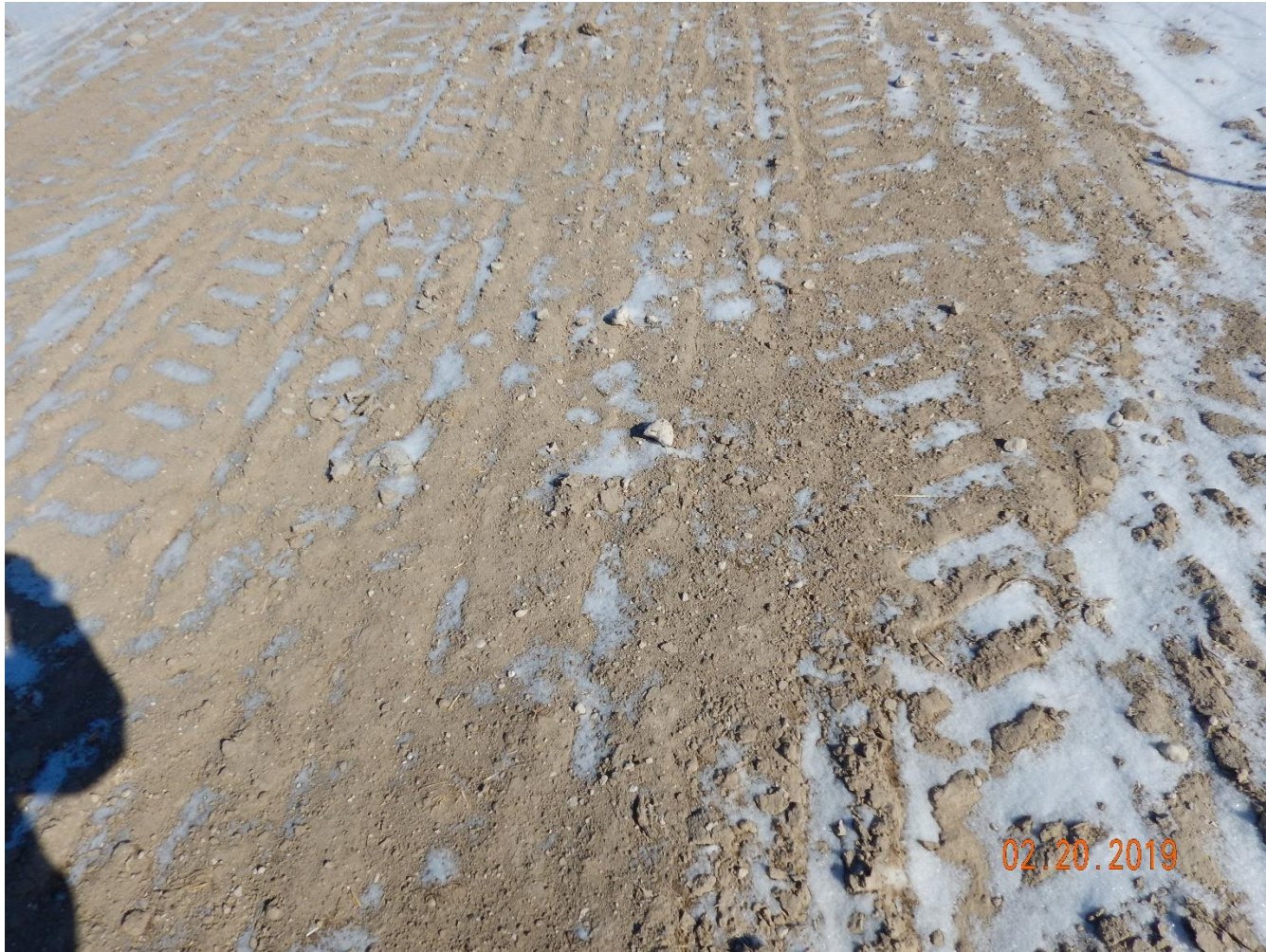
Photo 16: Photo taken from the disturbed interim areas on the west end of the pit. Photo shows the seeded soils of the interim areas remain bare and exposed. Previous inspections required stabilization control BMPs to stabilize the seeded soils to mitigate further erosion degradation. Unable to find evidence that stabilization controls have been installed/maintained; Areas downgrade of the pit and location remain at risk to erosion degradation.
