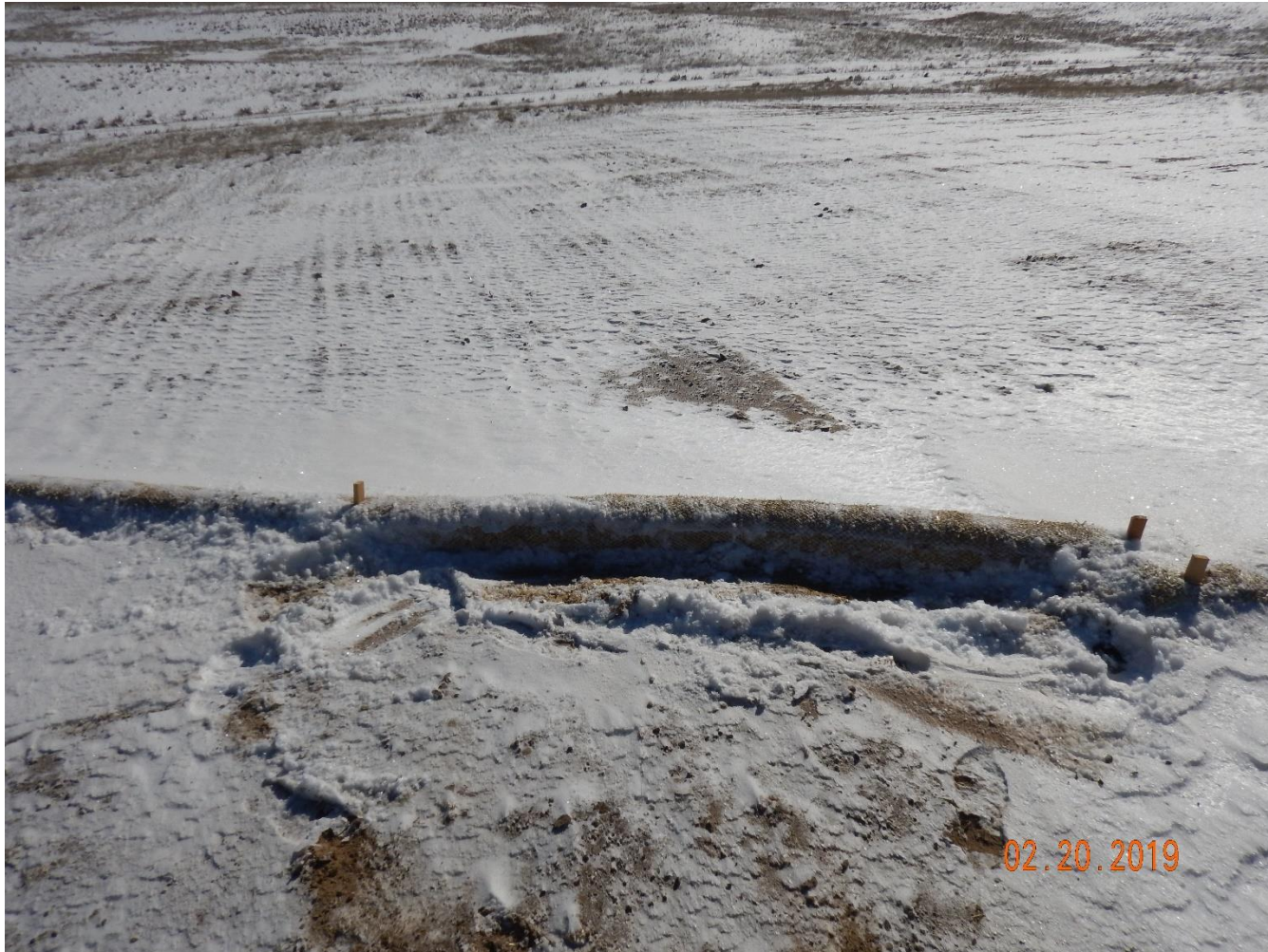
Photo 8: Continued from photo 7. Photo shows erosion log has not been trenched and backfilled in accordance with good engineering practices. See comments under photo 2. Photo also shows operator appears to have seeded with the contour of the slope, rather than along the contour. This is not advised as seed rows can concentrate stormwater flows down the slope and facilitate rill and gully erosion.
