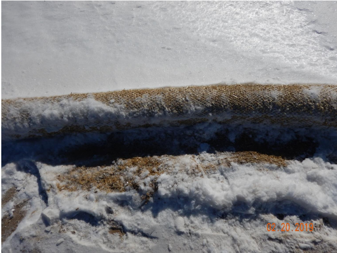
Photo 9: Continued from photo 8. Photo shows erosion log has not been trenched and backfilled in accordance with good engineering practices. See comments under photo 2
