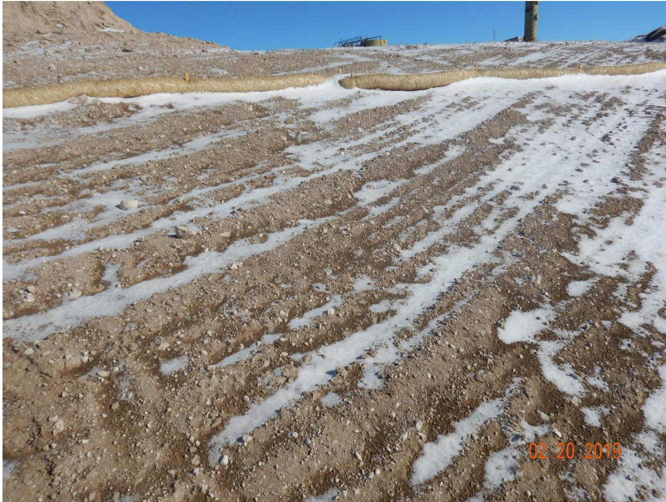
Photo 3: Photo taken from the disturbed interim areas on the east end of the pit. erosion log. Photo also show the seeded soils of the interim areas remain bare and exposed. Previous inspections required stabilization control BMPs to stabilize the seeded soils to mitigate further erosion degradation. Unable to find evidence that stabilization controls have been installed/maintained; Areas downgrade of the pit and location remain at risk to erosion degradation. Parallel striations observed in the soils are likely a result from seeding activities using a no-till drill and are not considered to be (or suitable as) a stormwater and erosion control BMP.
