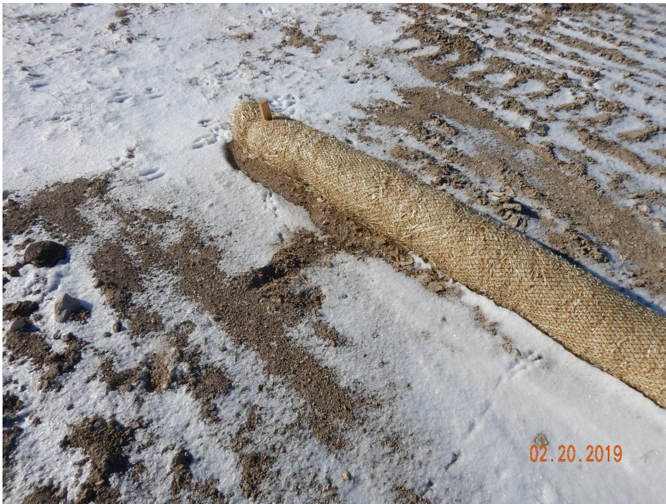
Photo 8: Continued from photo 7. Photo shows erosion log BMP. Erosion logs are sediment control barriers and ponding BMPs that intercept sheet flow runoff from disturbed areas, and are required to be trenched and back-filled in order to be in proper functioning condition. Photo shows Operator appears to have only placed/staked the erosion logs upon the surface of the soil; BMPs have not been trenched and back-filled in accordance with good engineering practices and are not in proper functioning condition.
