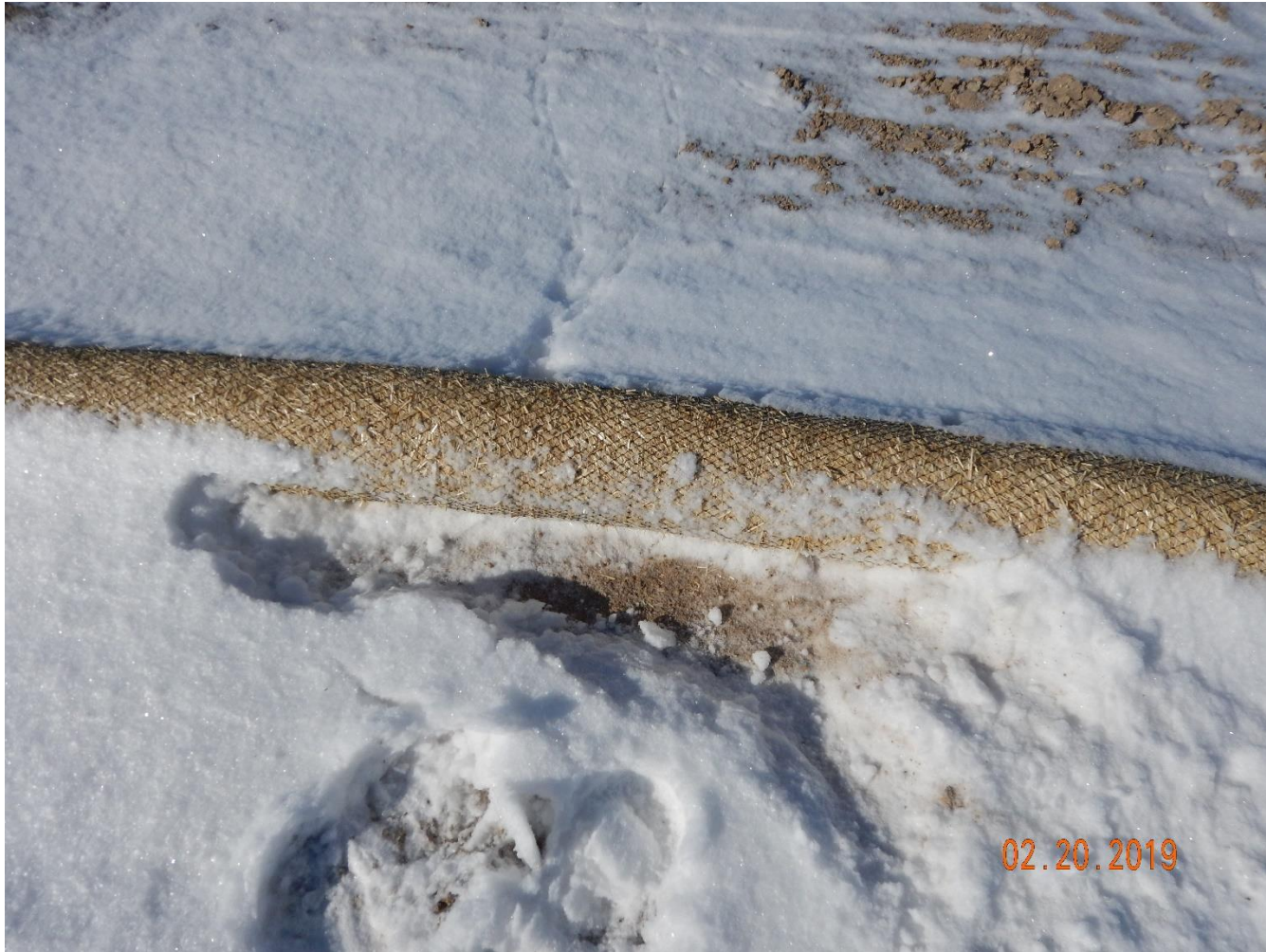
Photo 12: Continued from photo 11. Photo shows erosion log BMP. See comments under photo 8.
