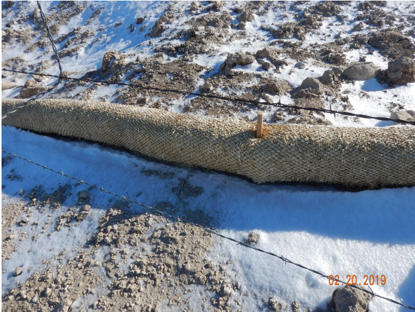
Photo 10: Photo taken from the base of the pit. Photo of erosion log. See comments under photo 8.
