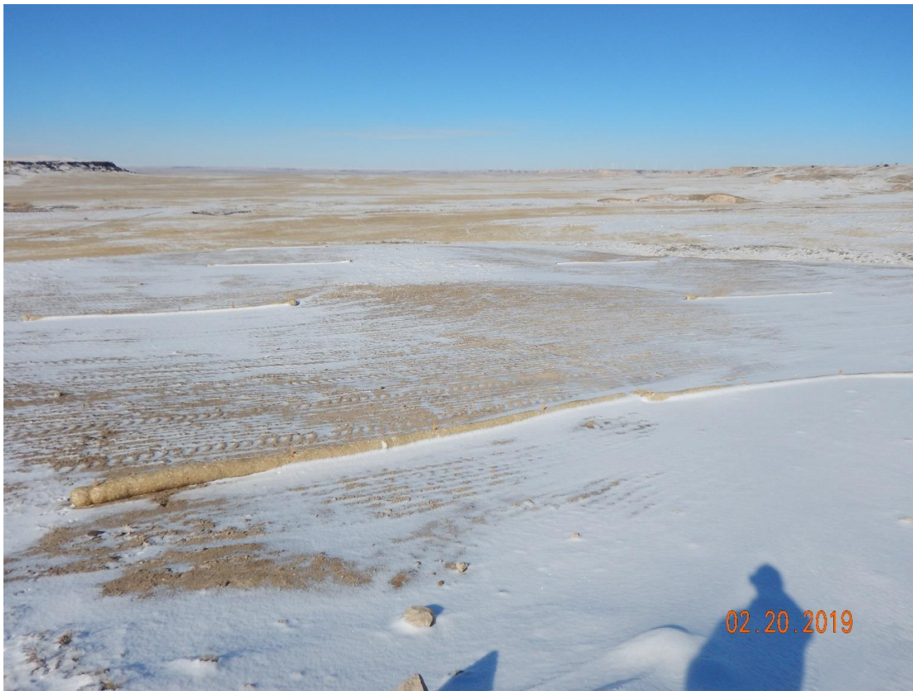
Photo 7: Photo taken from the west end of the production area/pit, facing west. Photo shows the disturbed areas down gradient of the pit and production areas. Photo shows operator appears to have placed erosion logs around the perimeter of the pit, and portions of the interim areas
