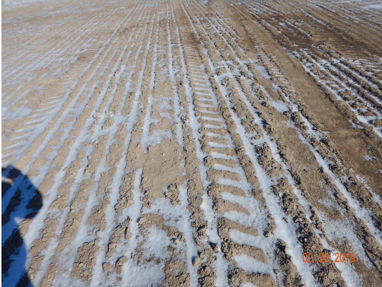
Photo 9: Photo taken from the interim areas west of the location. Photo shows the seeded soils of the interim areas remain bare and exposed. See comments under photo 3 regarding previous requirements for required stabilization controls.
