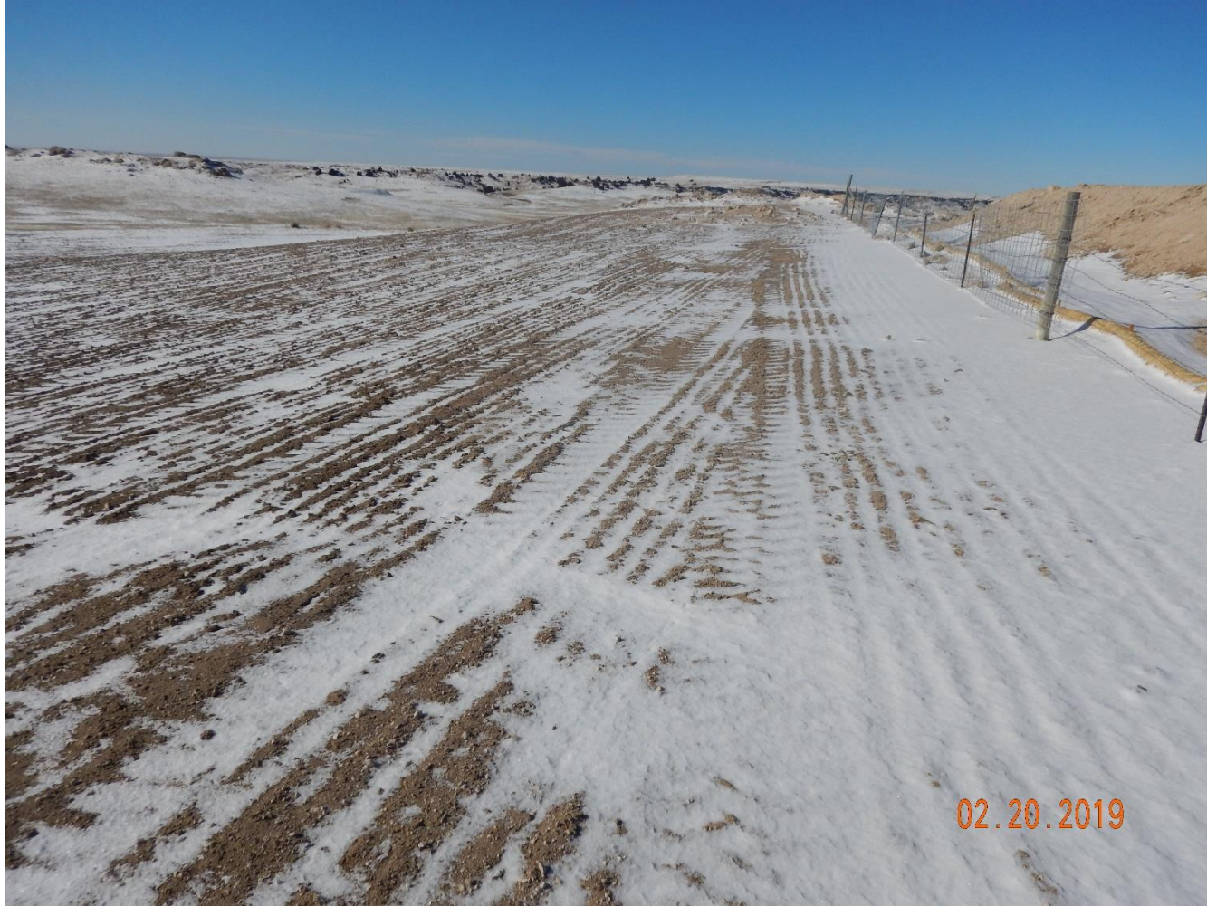
Photo 4: Photo taken from the interim areas on the south end of the pit, facing west. See comments under photo 3. Parallel striations observed in the soils are likely a result from seeding activities using a no-till drill and are not considered to be (or suitable as) a stormwater and erosion control BMP.
