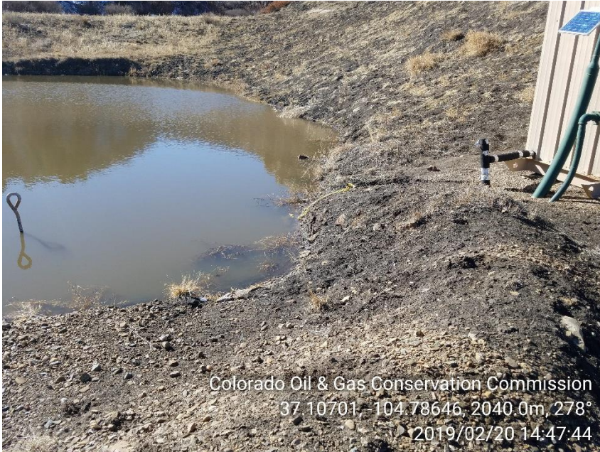
PHOTO 3: PRODUCED WATER LEVEL IN PIT IS ABOVE FREEBOARD MARKER
