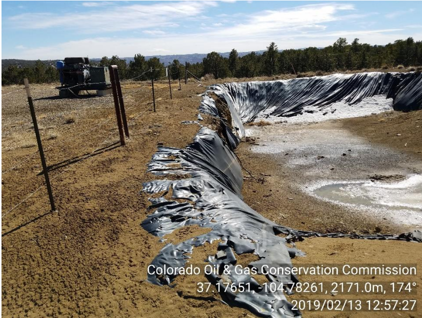
PHOTO 5: PRODUCED WATER PIT LINER IS TORN AND IN DISREPAIR
