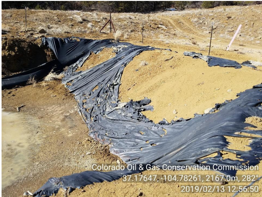
PHOTO 3: PRODUCED WATER PIT LINER IS TORN AND IN DISREPAIR
