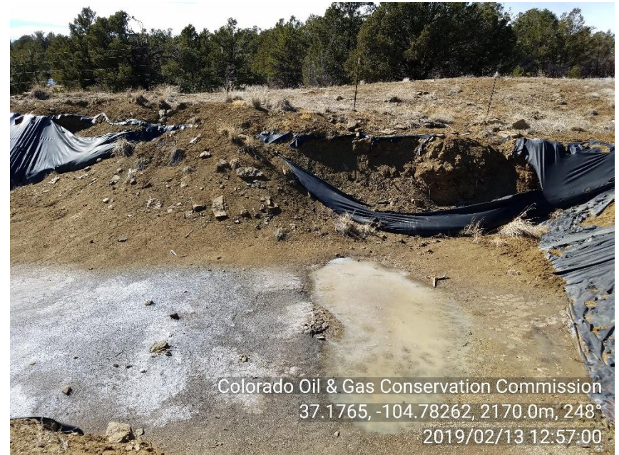
PHOTO 4: PRODUCED WATER PIT LINER IS TORN AND IN DISREPAIR
