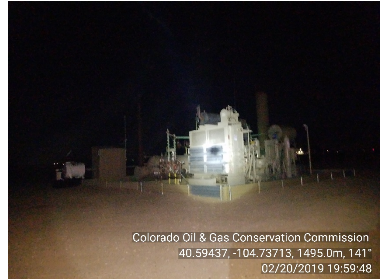
Compressor at battery (suspected noise source)
