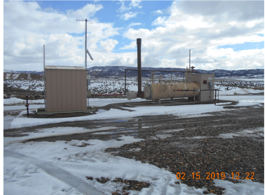
Meter housing and Separator
