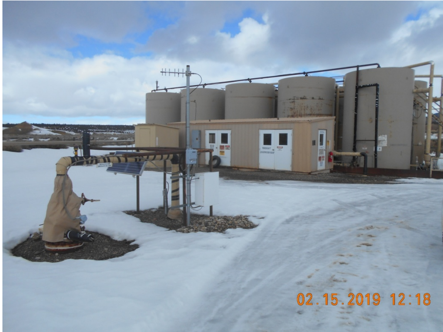
Injection wellhead, pump housing and tank battery
