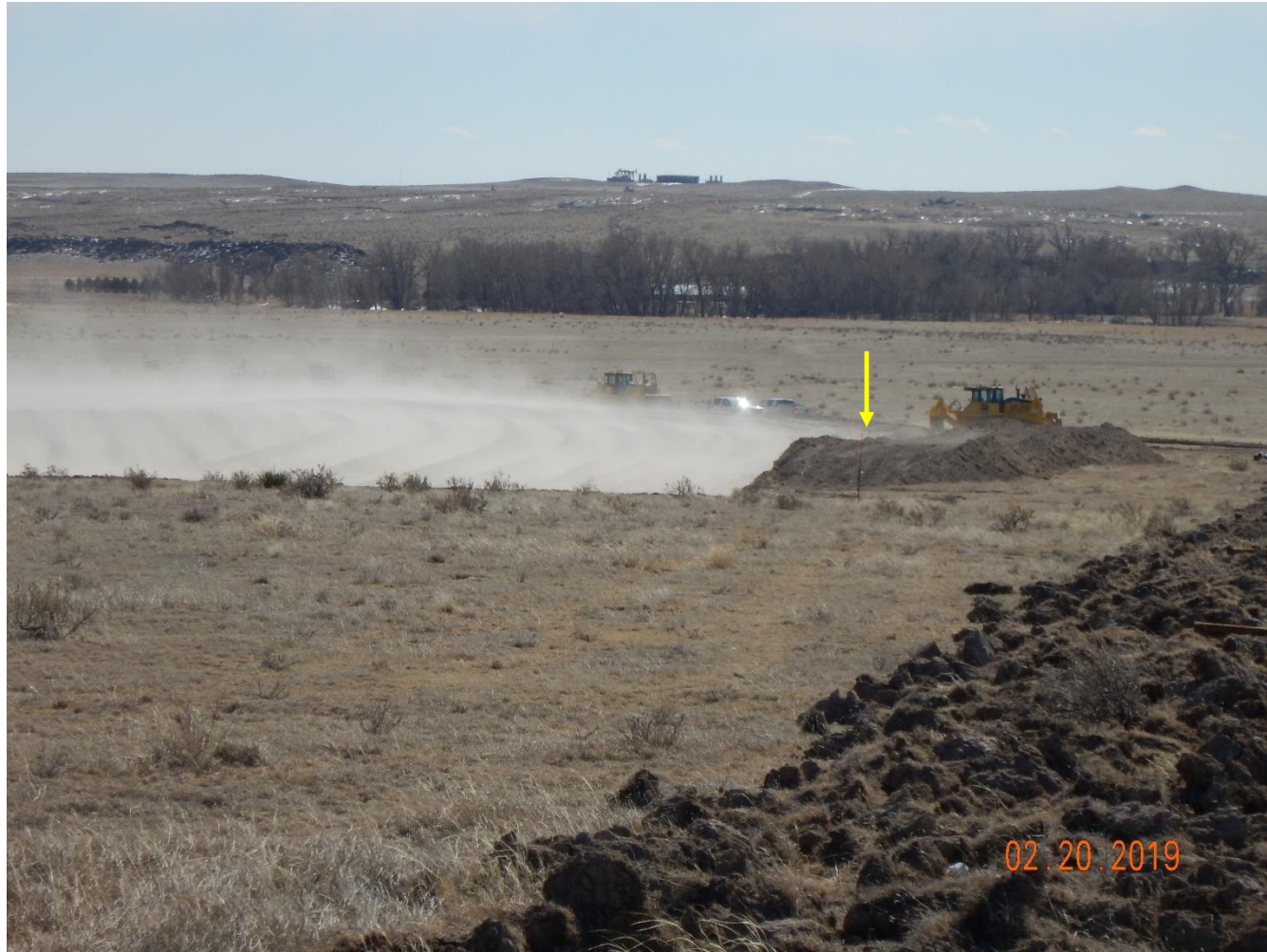
Photo 7: Photo taken from the west end of the location, facing south. Photo shows ongoing wind erosion transporting sediment offsite from an un-stabilized soil stockpile (arrow). This does not comport with rule 1002.e and 1002.f
