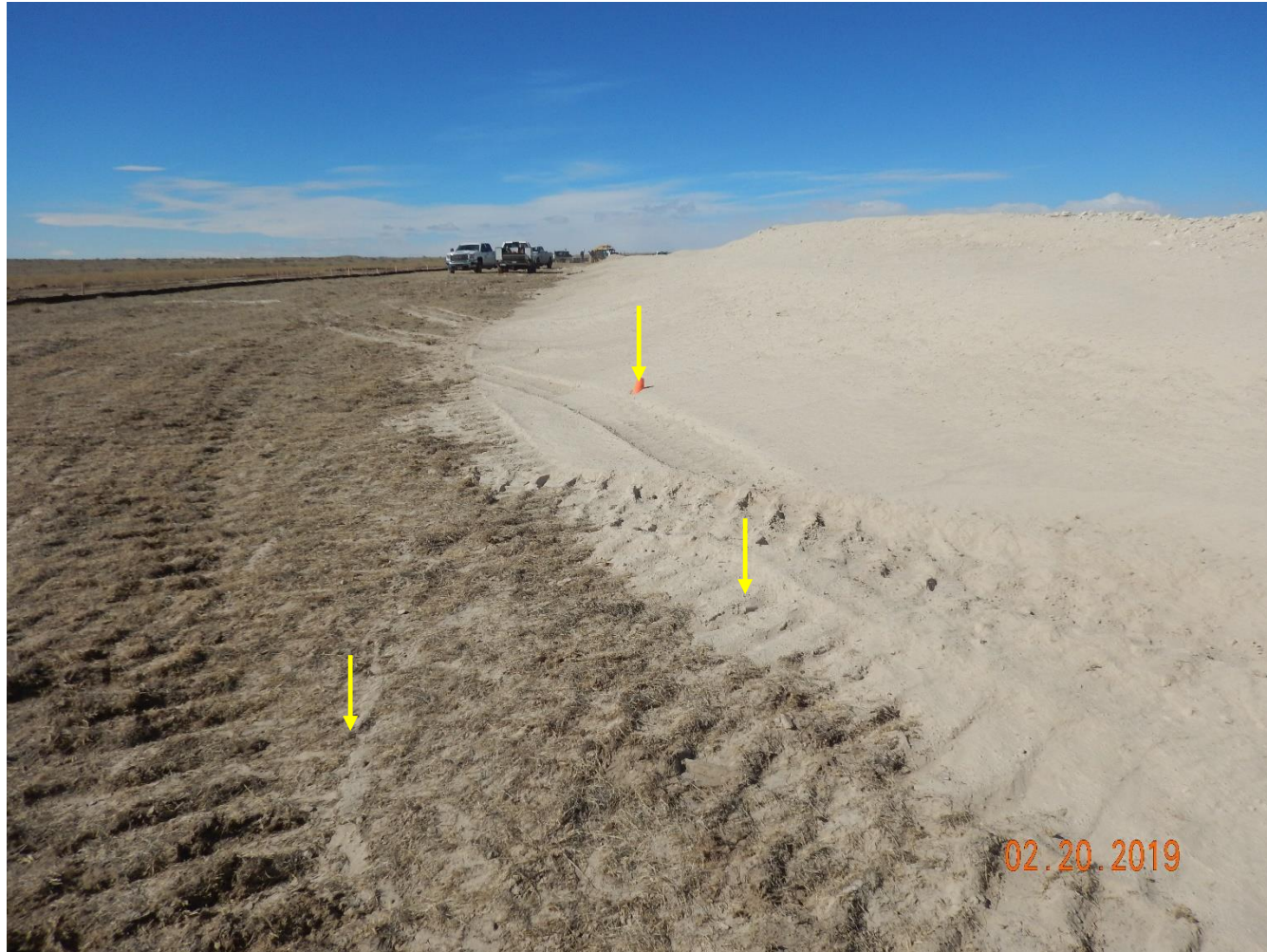
Photo 25: Photo taken from the southwest end of the location, facing northwest. Photo shows sediment deposition from the pad appears to have almost covered an orange cone. Photo also shows sediment transport and deposition from the pad
