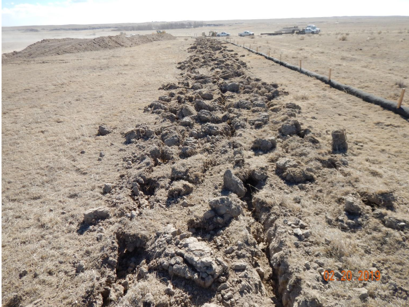
Photo 5: Photo taken from the west end of the location. Photo shows operator has implemented surface roughening as a perimeter stormwater BMP. Surface roughening is a temporary BMP that should be used in conjunction with other BMPs.
