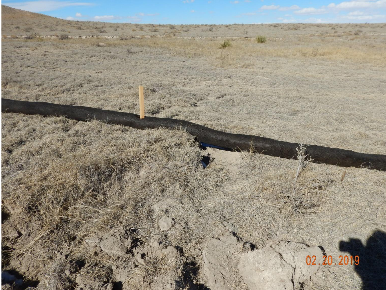
Photo 9: Photo taken from the north end of the location, facing north. Photo shows operator has implemented a “Filtrexx” perimeter control wattle BMP. Based on site conditions (topography), BMP does not appear to be sufficient; BMP does not achieve a 100% soil surface contact, or appear to have the weight to mitigate stormwater runoff and allow for stormwater ponding without trenching and backfilling. Photo shows one example of areas observed on location where BMP has not achieved sufficient soil surface contact.
