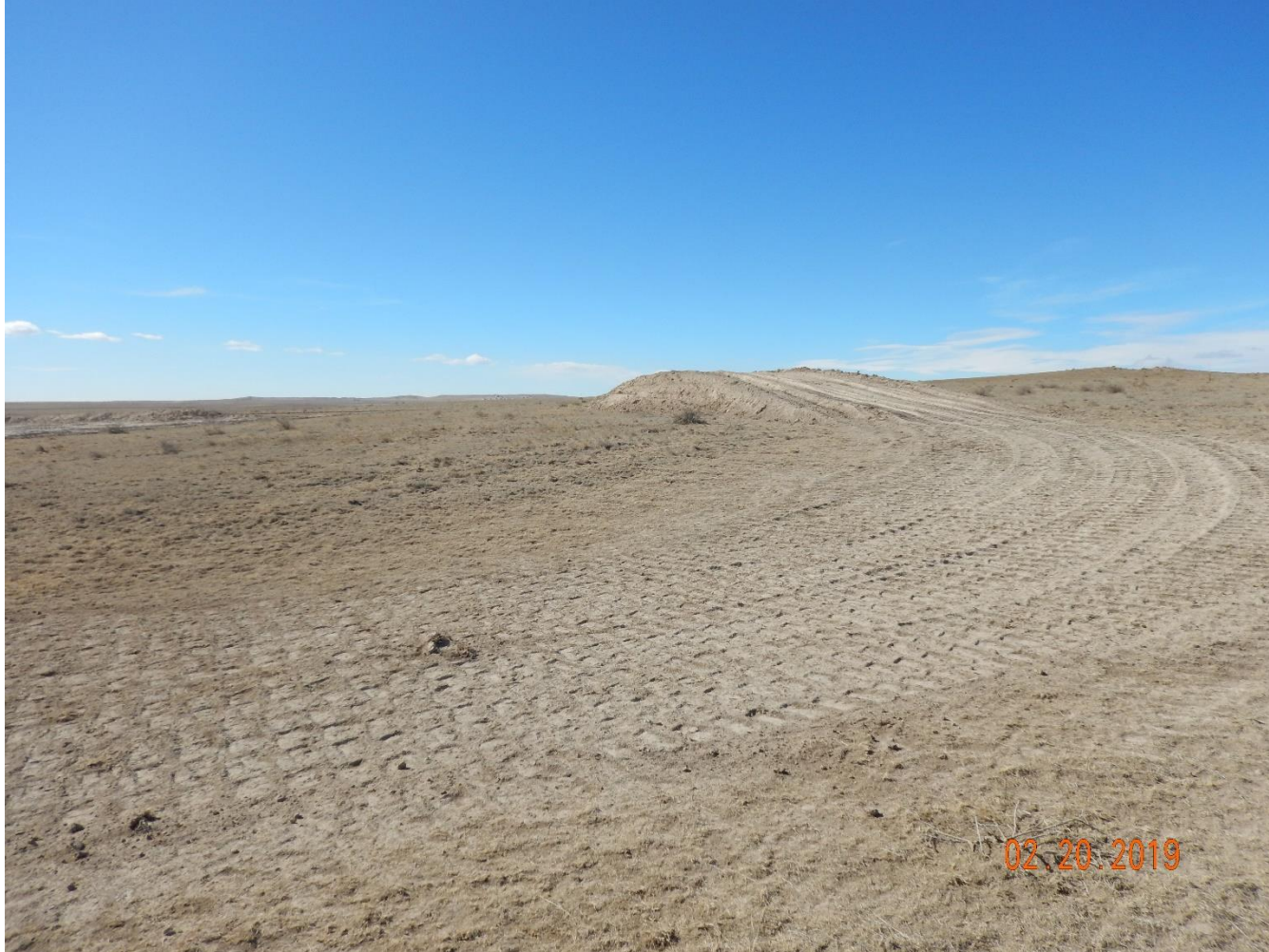
Photo 12: Photo taken from the east end of the location, facing west. Photo shows one of the soil stockpiles for the location. Soil stockpile has not been sufficiently stabilized, is currently loose material and at risk to erosion degradation.
