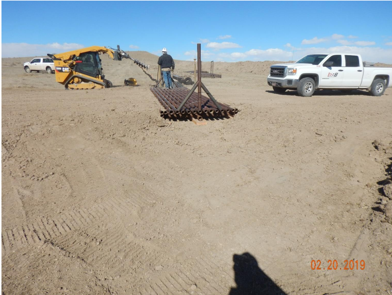
Photo 28: Photo taken from the southwest corner of the location. Photo shows workers installing a cattle guard on the site.
