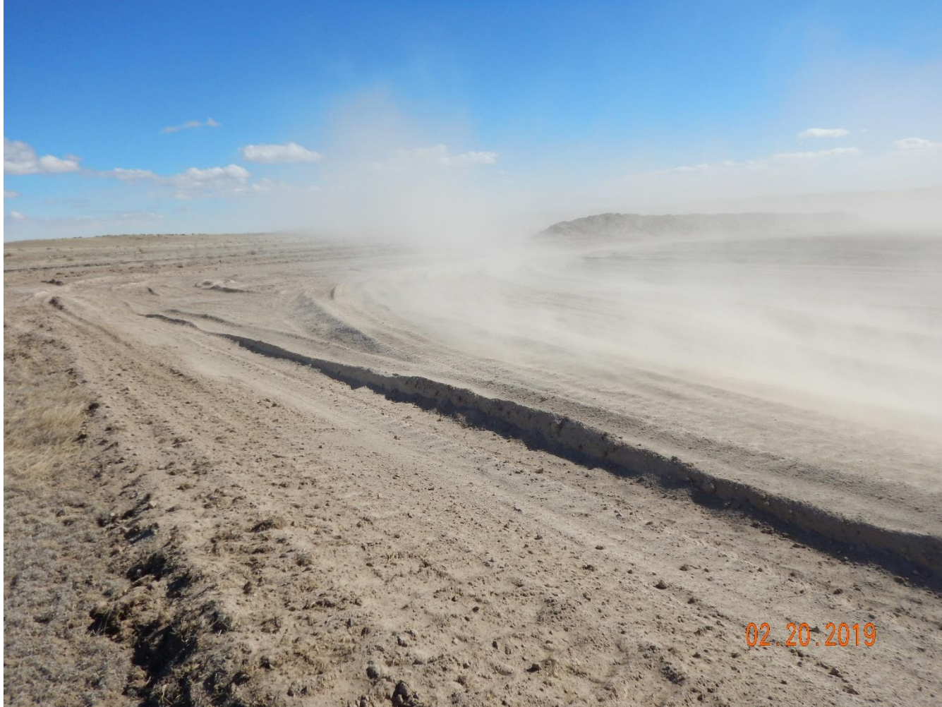
Photo 14: Photo taken from the north end of the disturbance area, facing east. Photo 14-16 shows overview of the current disturbance area from east, to south, to west. Photos also show ongoing wind erosion transporting sediment offsite. This does not comport with rule 1002.e and 1002.f
