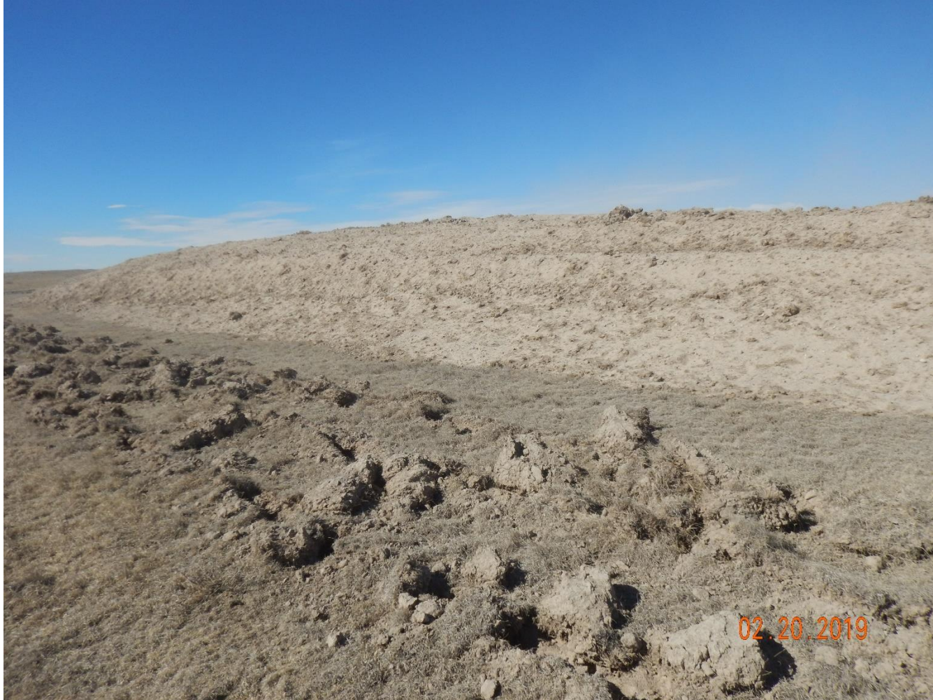
Photo 21: Photo taken from the south end of the location. Photo shows topsoil stockpile. Soil stockpile has not been sufficiently stabilized, is currently loose material and at risk to erosion degradation.
