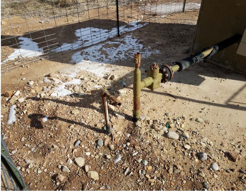
Location Photo #3, Unmarked/unused flow line riser.
