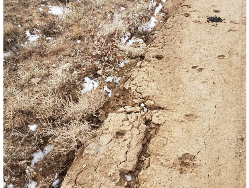
Location Photo #8, Rilling occurring along access road.
