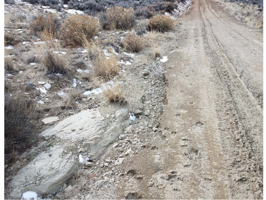
Location Photo #2, Rilling occurring along access road.
