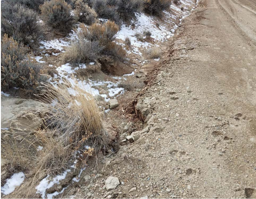
Location Photo #3, Rilling occurring along access road.
