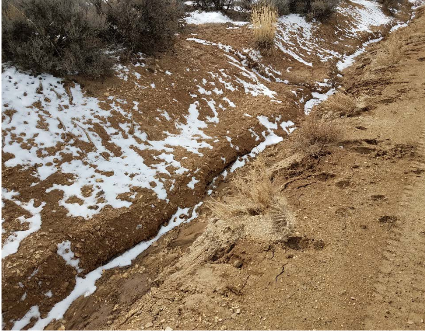
Location Photo #5, Rilling occurring along access road.
