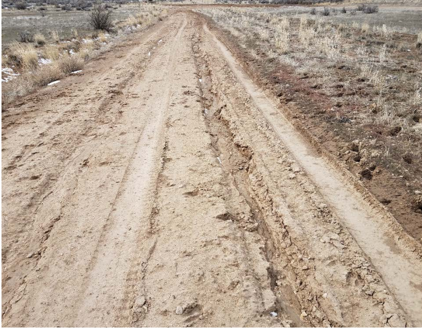
Location Photo #7, Rilling occurring along access road.
