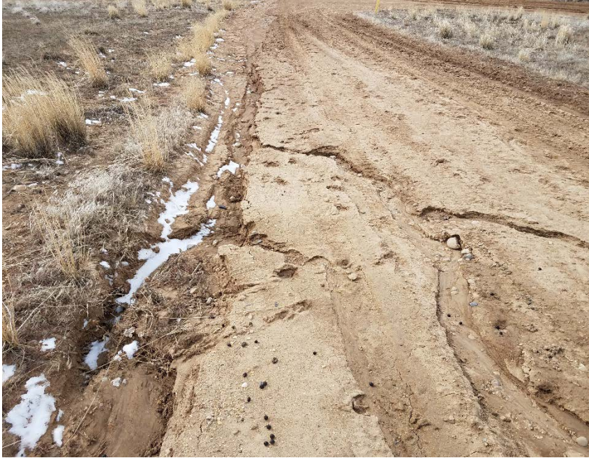
Location Photo #9, Rilling occurring along access road.
