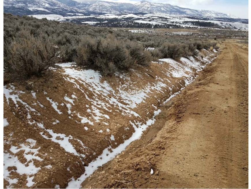
Location Photo #4, Rilling occurring along access road.
