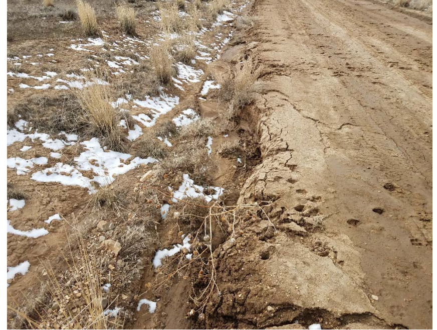
Location Photo #6, Rilling occurring along access road.
