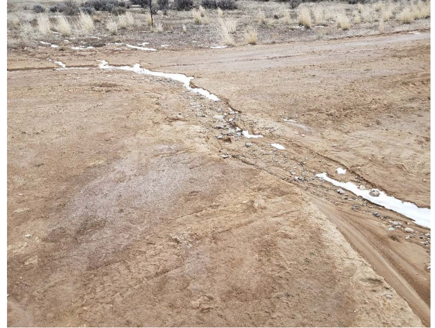
Location Photo #10, Sediment being moved across road.
