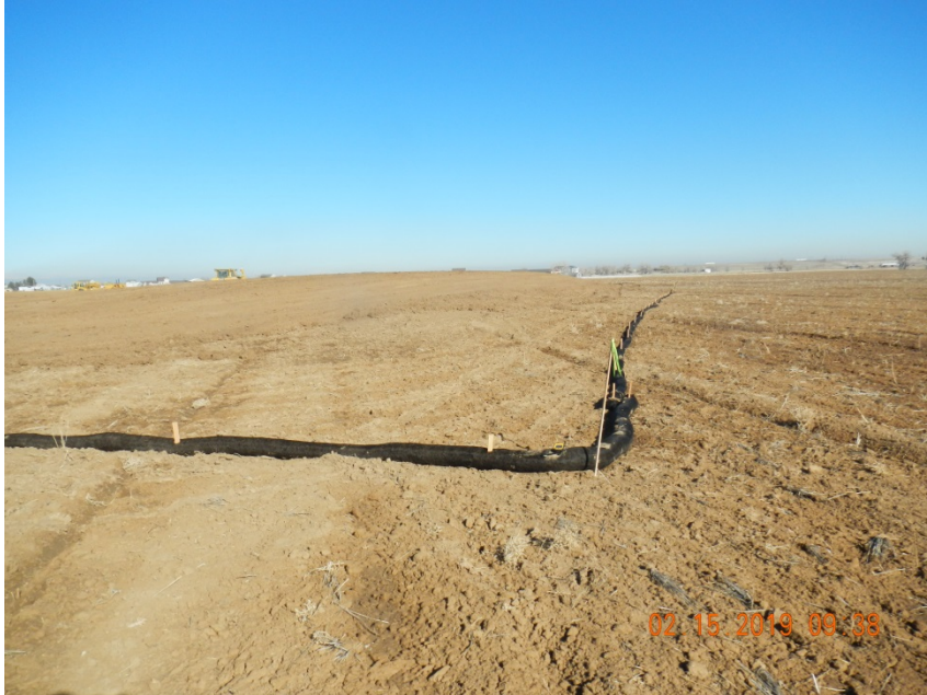
Photo 3. Photo taken from the southeastern perimeter of the location, facing North. Photo illustrates a filter strip BMP that has been installed around the entire perimeter of the location in conjunction with other BMPs.
