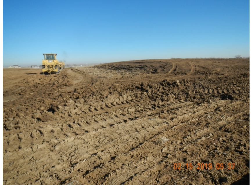
Photo 2. Photo taken from the location, facing West. Photo illustrates the topsoil stockpile being stored along the eastern area and has been temporarily stabilized with equipment tracking.
