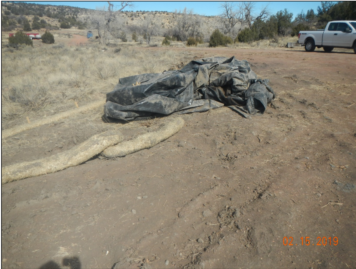
Photo 4. Plastic liner debris remains on the side of the access road. Wattles are displaced and not properly installed. Connection between the wattles were not properly overlapped.
