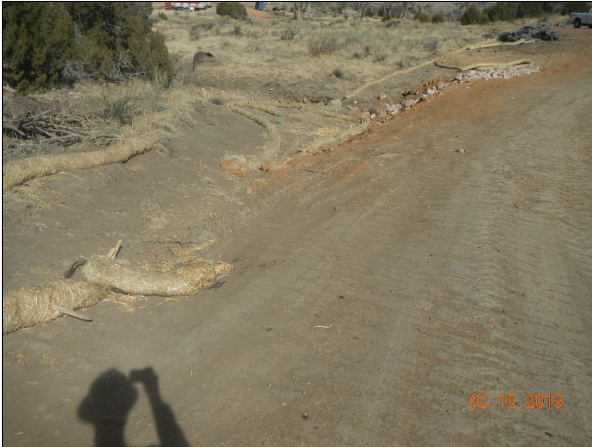
Photo 8. The wattles are displaced and improperly installed along the access road.
