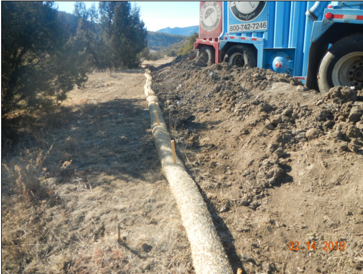
Photo 11. Facing south along the east side of the location. Loose soil is pushed up covering the berm and can potentially overtop the wattles. There is no tertiary containment along the down gradient parameters of the location. Connection between the wattles were not properly overlapped.
