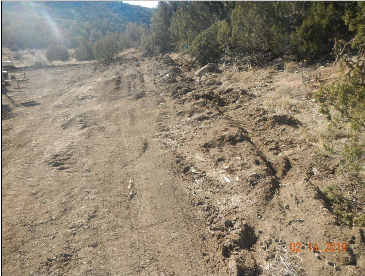
Photo 14. The ditch along the west side of the location is not properly installed. The gradient of the ditch will drain water toward this low area allowing stormwater to flow onto the pad. Ditch is not properly excavated in this area.
