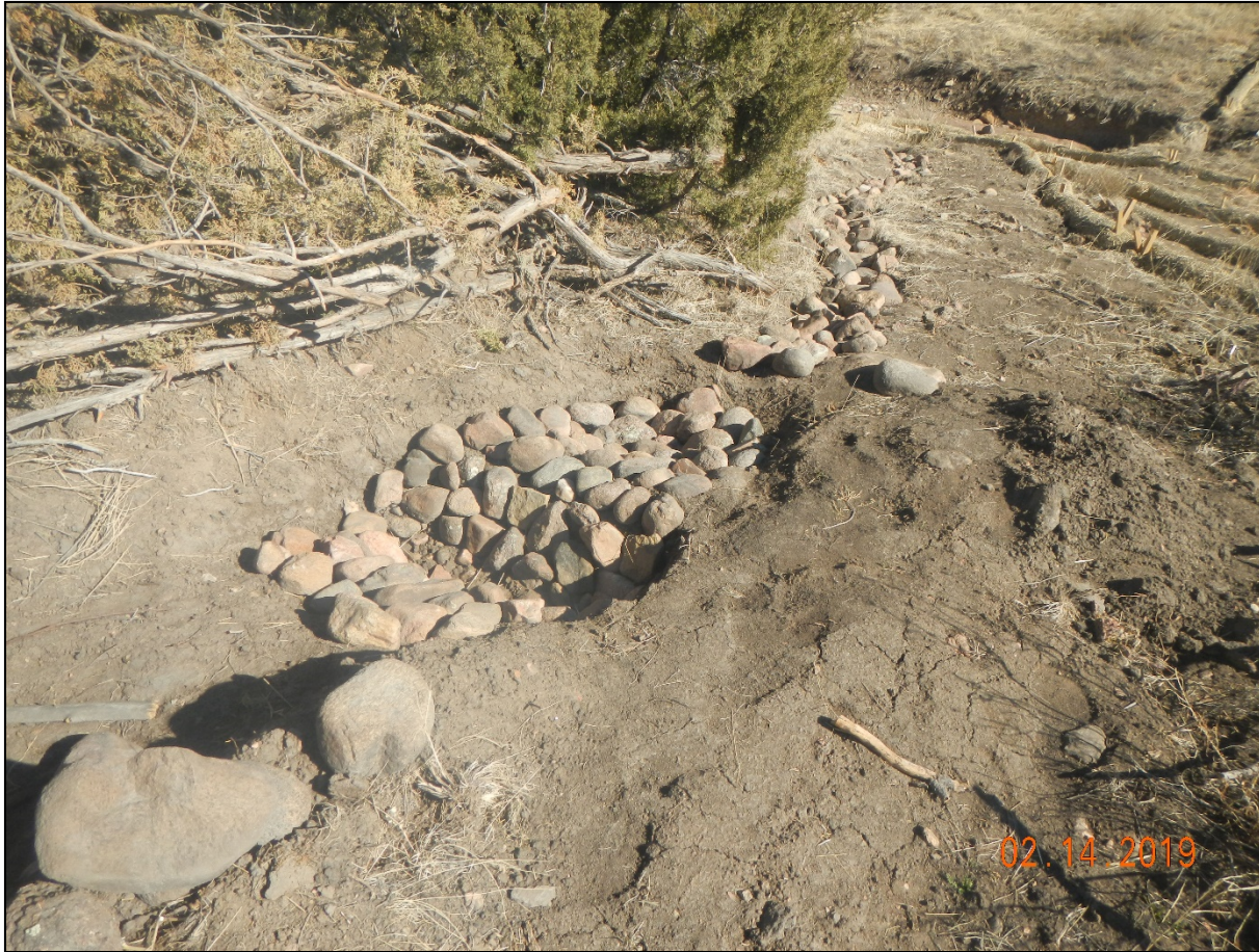
Photo 17. Sediment trap at the north side of the location is drastically undersized to handle runoff. Dimensions are 4'L x 3'W x 2'depth.
