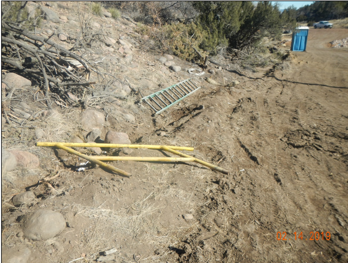
Photo 16. Various equipment debris lay's along the stormwater ditch. The ditch is not properly excavated in this area.
