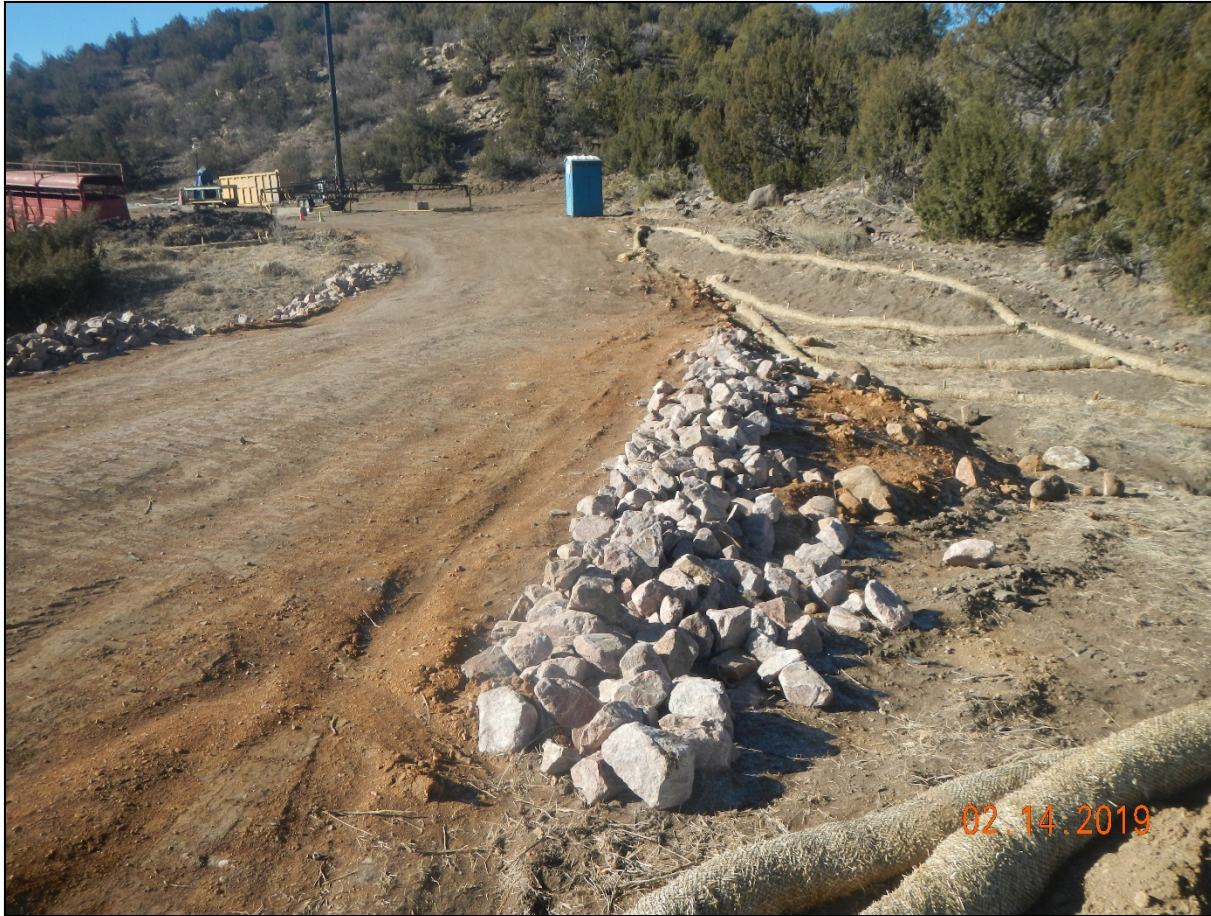
Photo 5. Facing southwest along access road toward the location. The road crosses the stream at this point. The stream crossing is inadequate.
