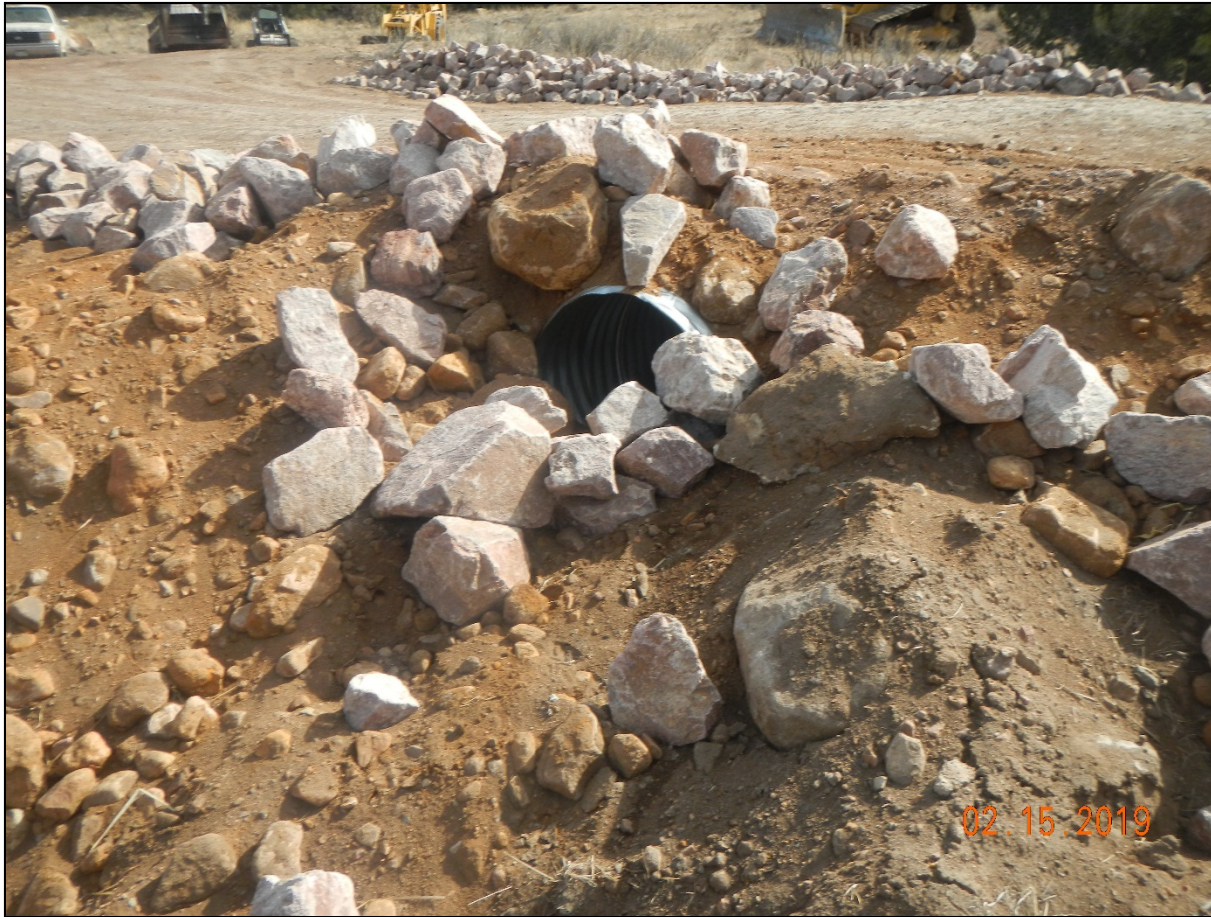
Photo 6. The outlet culvert at the stream crossing is obstructed with material and is improperly installed (See Photo 7).
