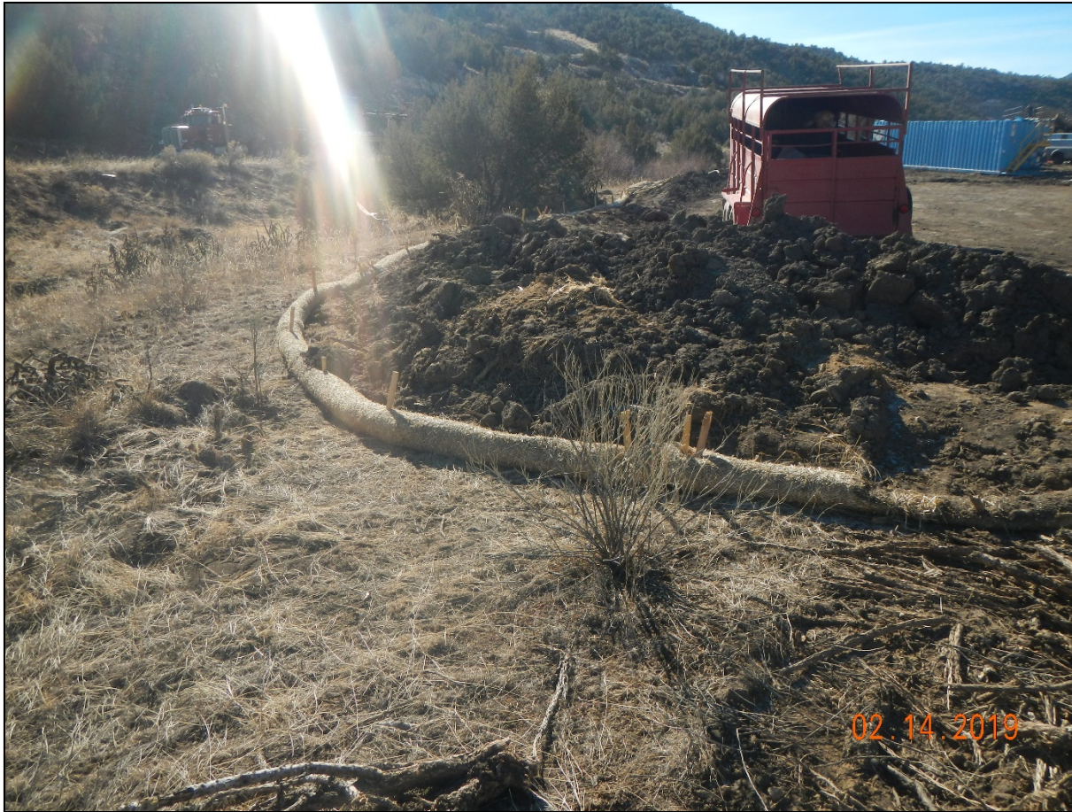
Photo 10. Wattles are placed along the eastern side of the location. Loose soil is pushed up covering the berm and can potentially overtop the wattles. There is no tertiary containment along the down gradient parameters of the location.
