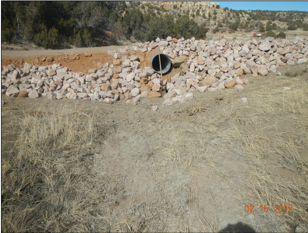
Photo 7. The inlet culvert at the stream crossing appears to be installed too high above the channel which will create pooling of the water and potential water overflow across the access road. This also shows improper installation and armoring.
