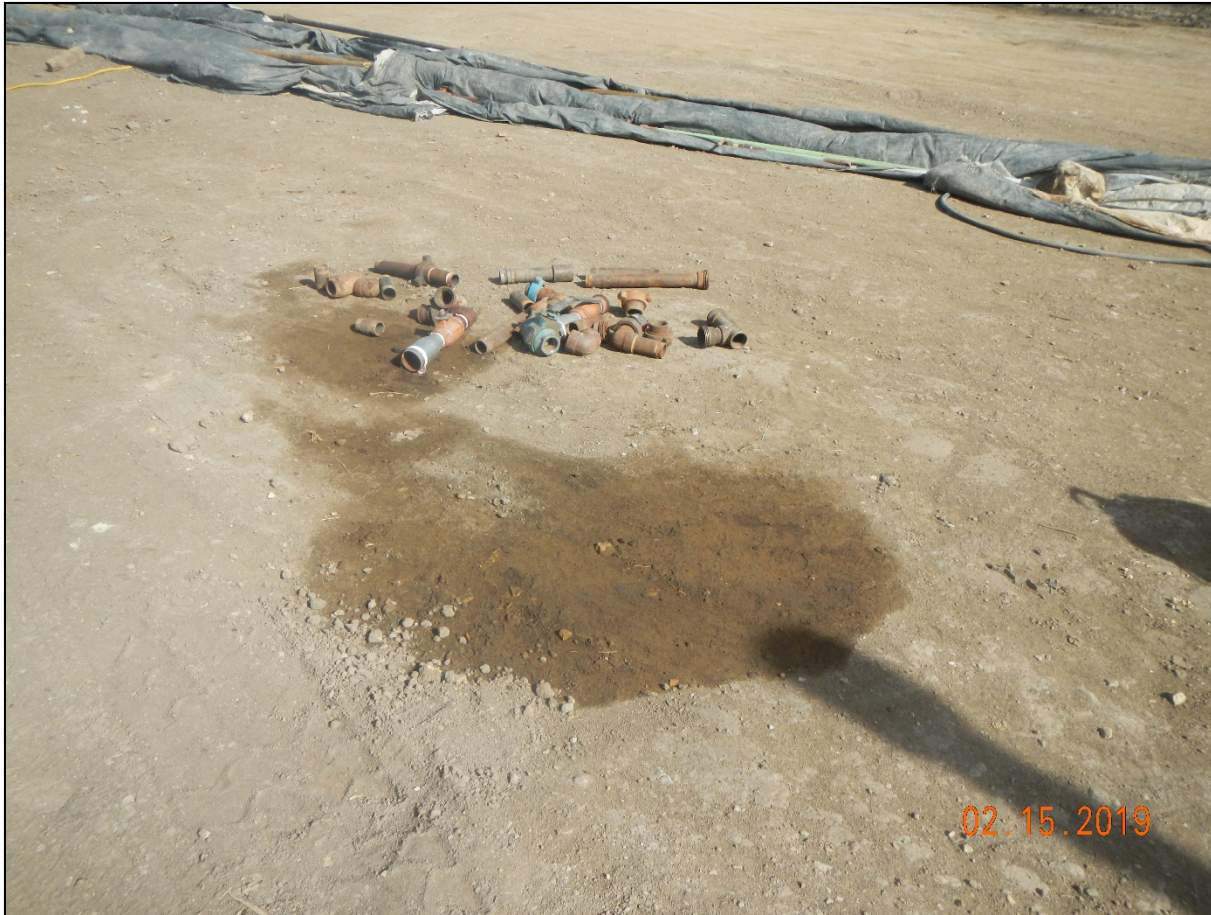
Photo 15. Oil stained soil was found near the wellhead approximately 3'x3' area. Various pipe fittings are left in this area.
