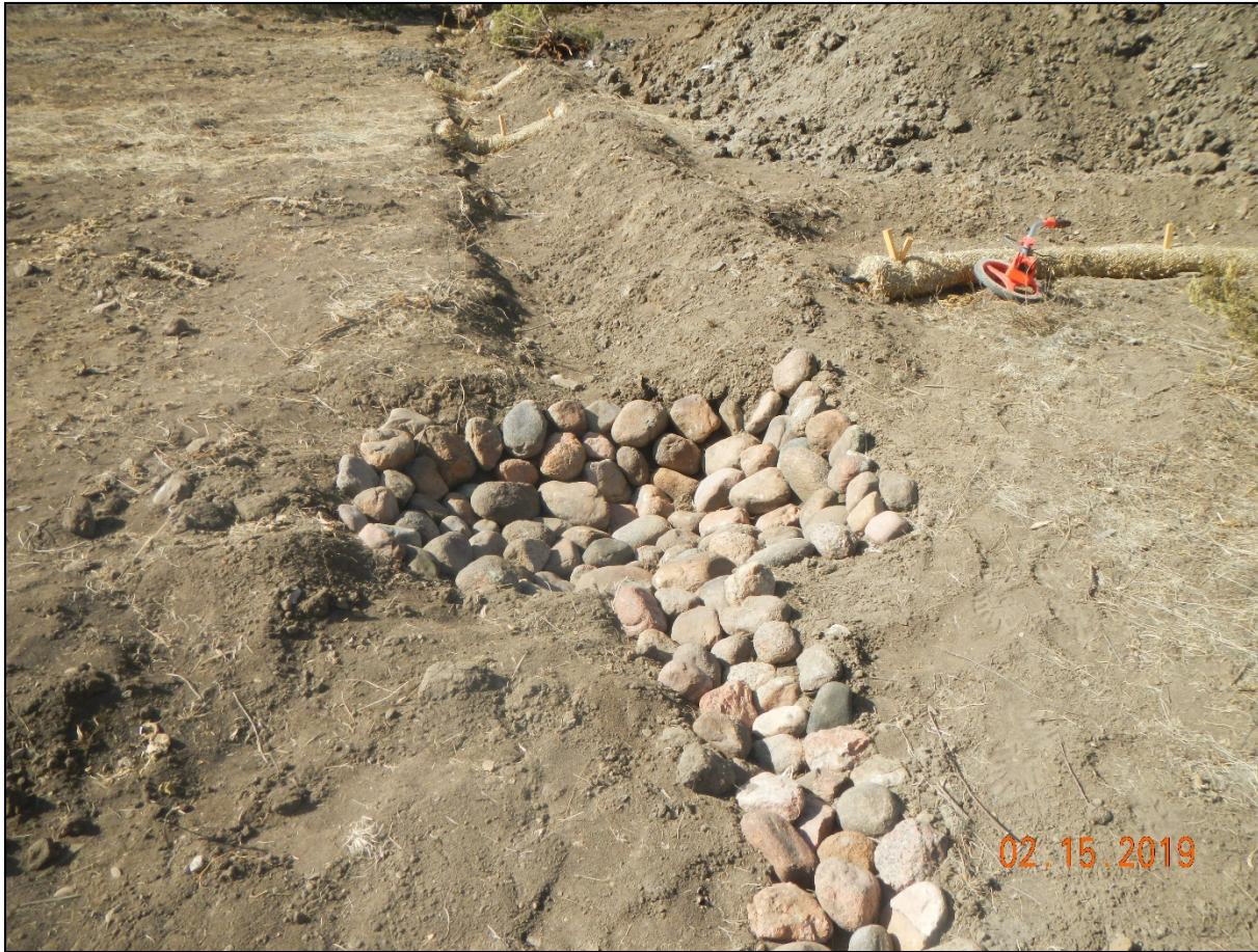
Photo 12. Sediment trap at the southeast corner of the location is drastically undersized to handle runoff. Dimensions are 5'L x 4'W x 2'depth.
