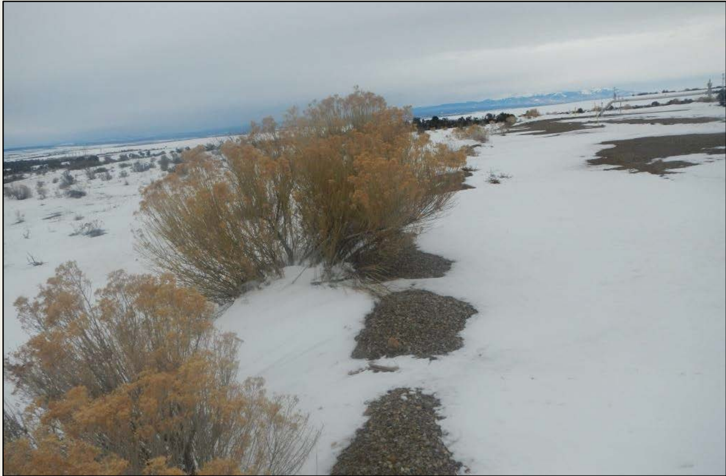
Photo 1. View of the northern project area from the northwestern corner facing eastward. Berm appears to be functioning.
