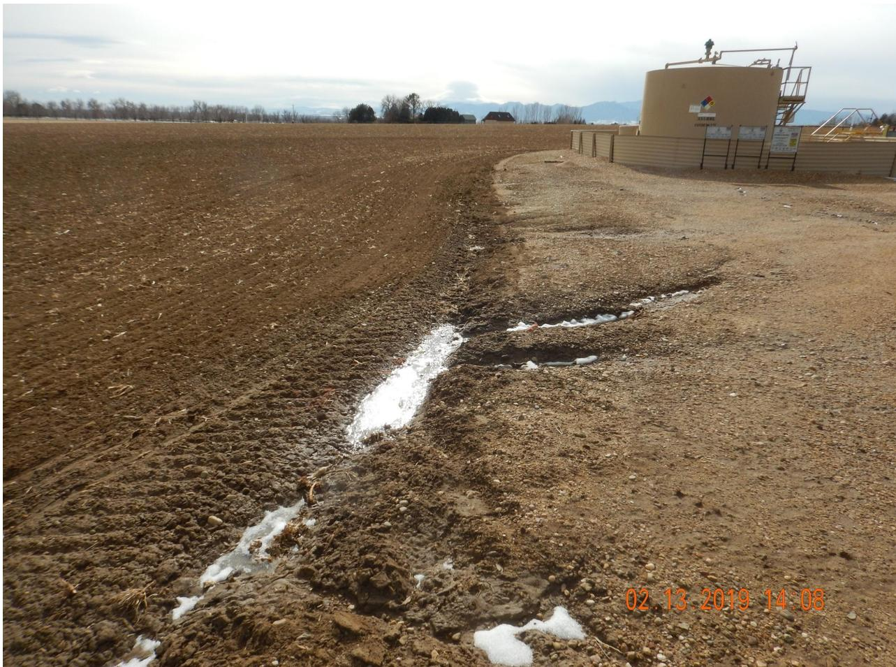
**Photo 1.** Photo taken from the production/well location, facing Southwest. Operator has failed to stabilize production areas per Rule 1003.b. Photo illustrates erosion along the perimeter of the production area.
