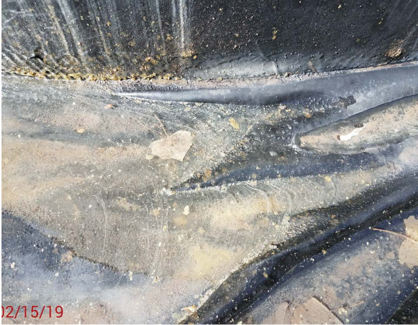
Location Photo #7, free floating condensate in battery containment.
