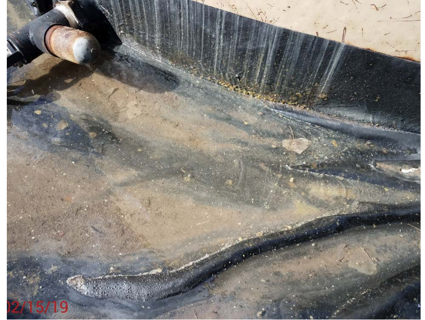
Location Photo #6, free floating condensate in battery containment.
