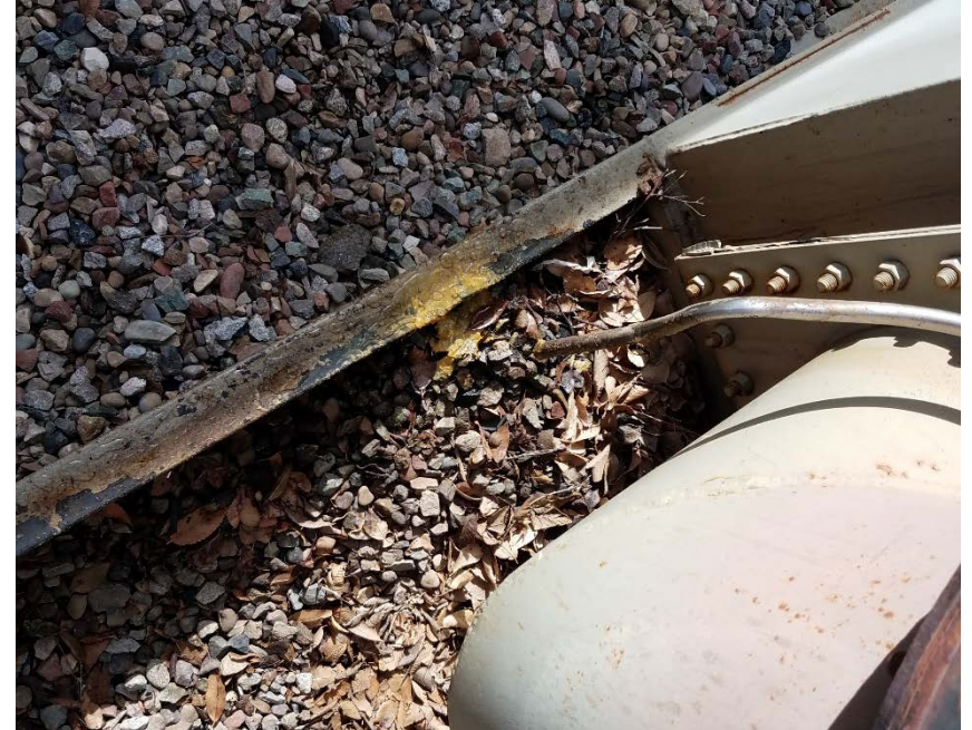
Location Photo #4, Stained ground at blow down at separator.
