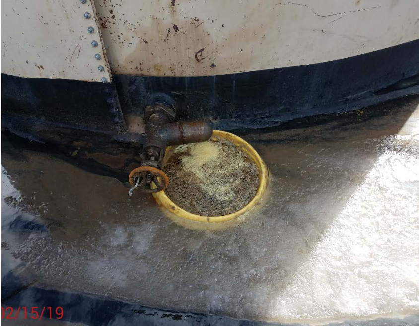
Location Photo #5, Condensate in drip pan.
