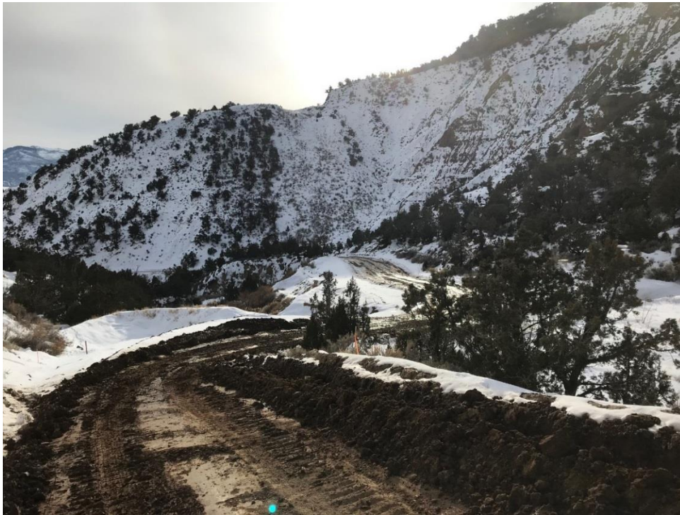
Photo 1. Narrow, steep, and curving access road leading to the DOE 1-M-18 well pad. Surveyed 20%
