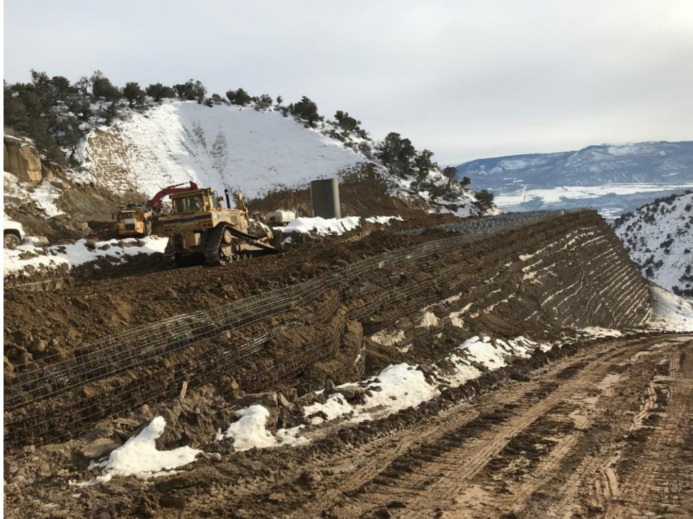
Photo 2. Preparing the DOE 1-M-18 well pad.
