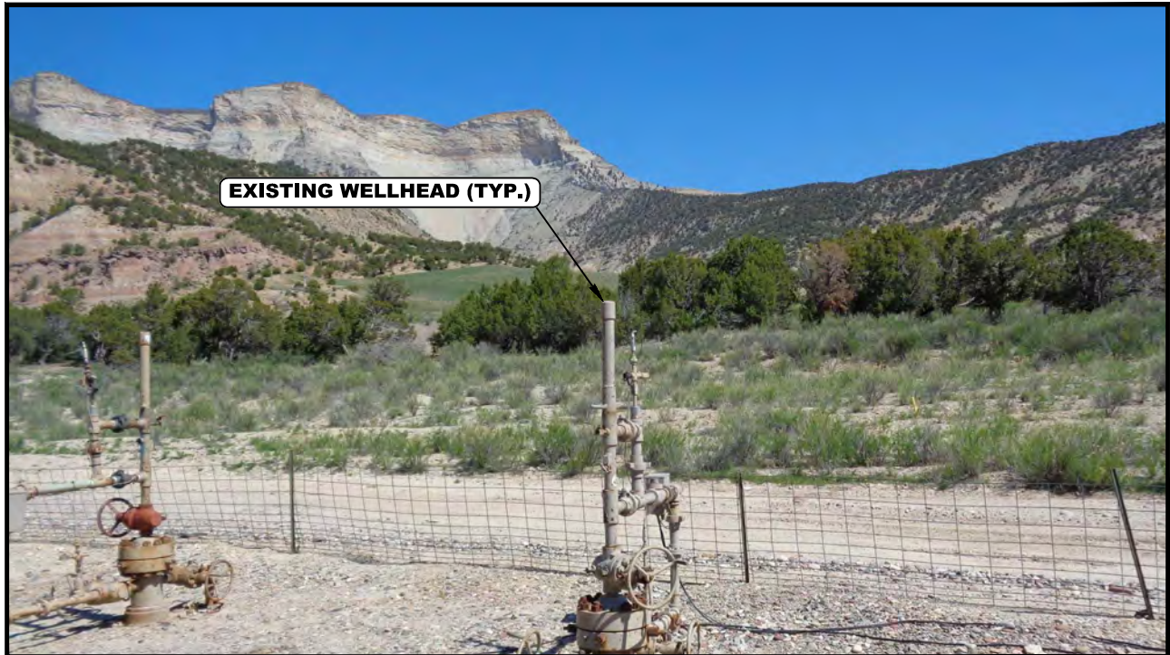
PHOTO: VIEW OF WELLHEADS
