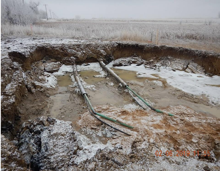
Bulthaup 16-6 and 39-6 flowlines exposed in excavation; The 39-6 flowline (failed) is furthest right. Flowlines enter 4" casing pipe under marshy area. View south to wellheads.
