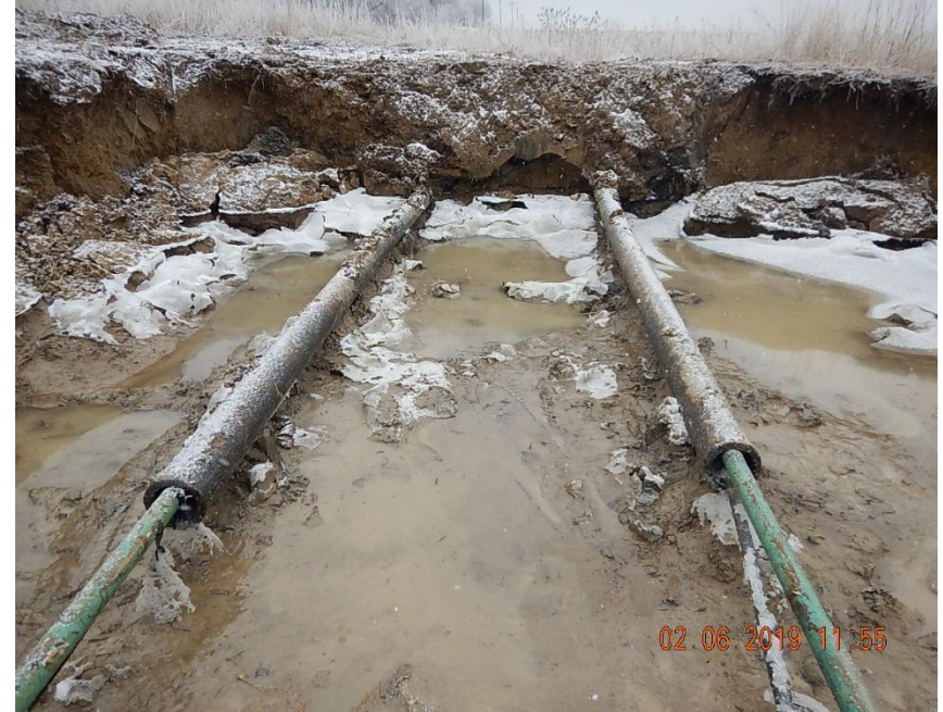
Closer view of the 2" FBE CS flowlines and 1" HDPE gas supply/ return flowlines entering the 4" steel casing pipes
