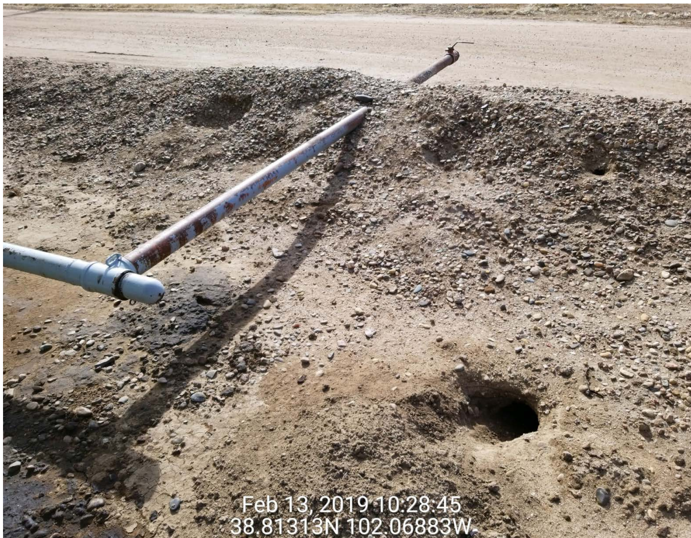
Rabbit burrow in tank battery containment wall.
