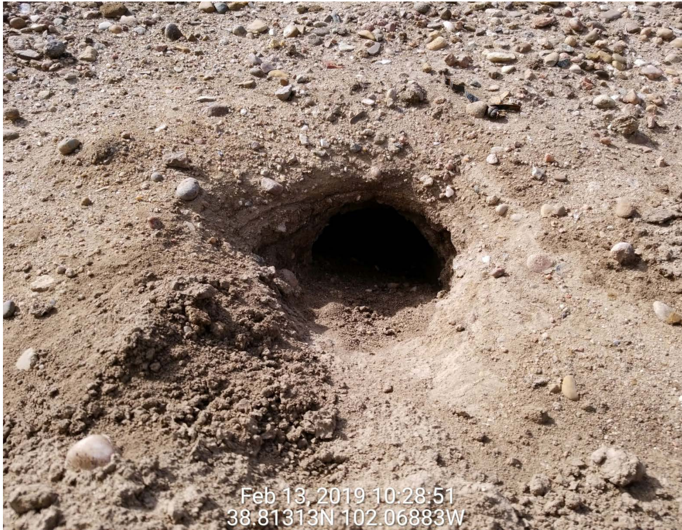
Rabbit burrow in tank battery containment wall.
