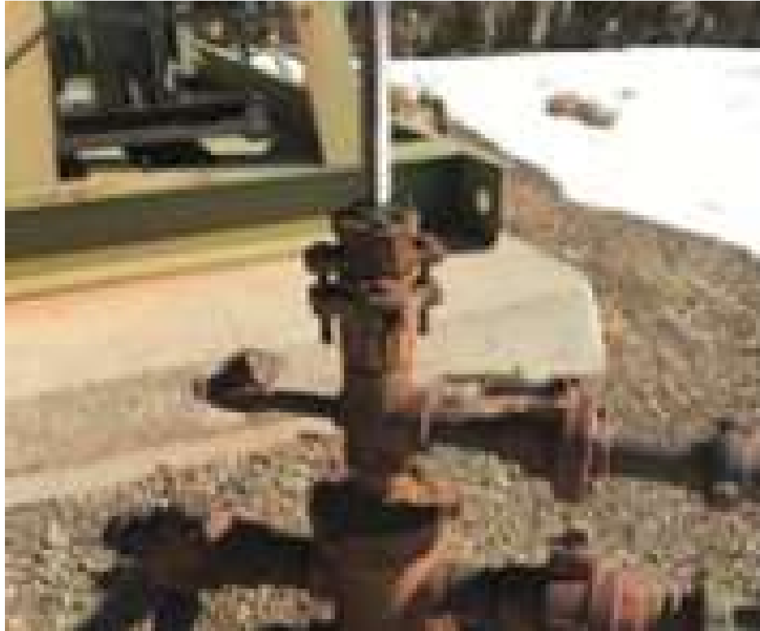
PHOTO 1: REPLACED PACKING TO ELIMINATE THE WATER LEAK.
