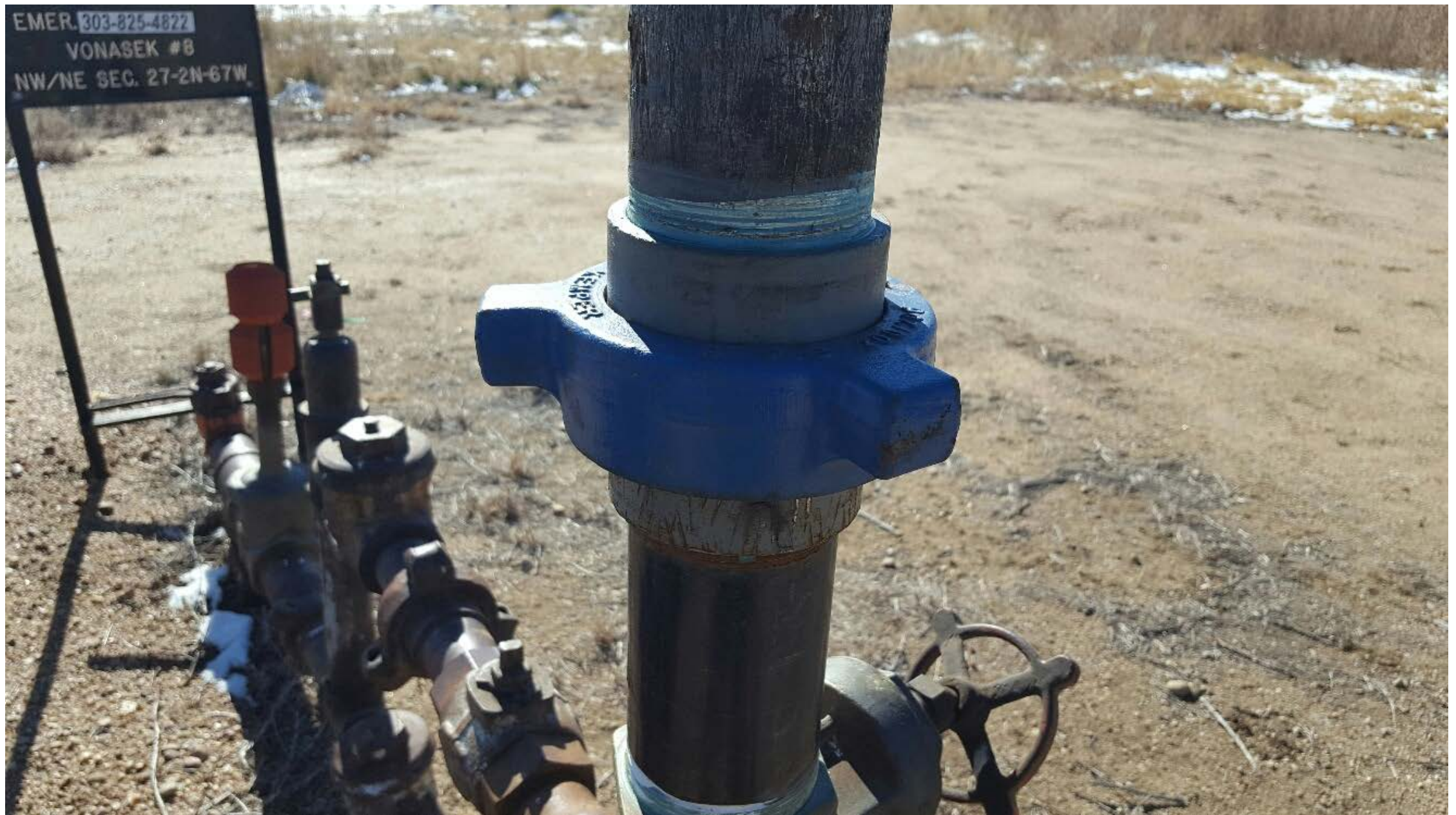
Figure #1 Hammer union has been replaced.
