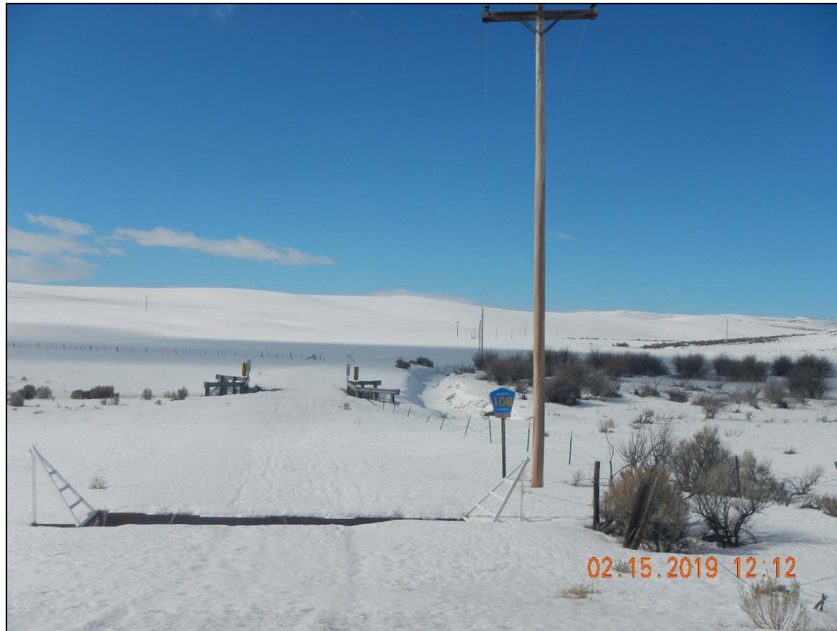
Photo 1. Overview of location taken at access road where maintenance stops.
