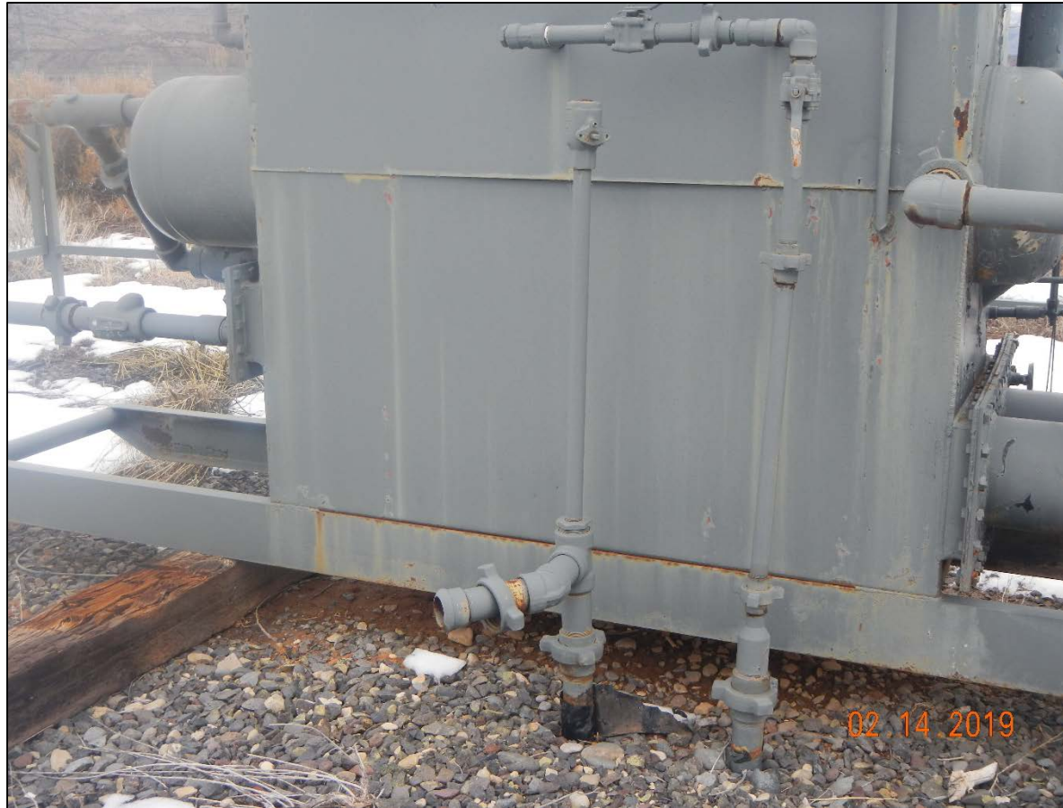
Unused, unmarked, locked out tagged out riser
