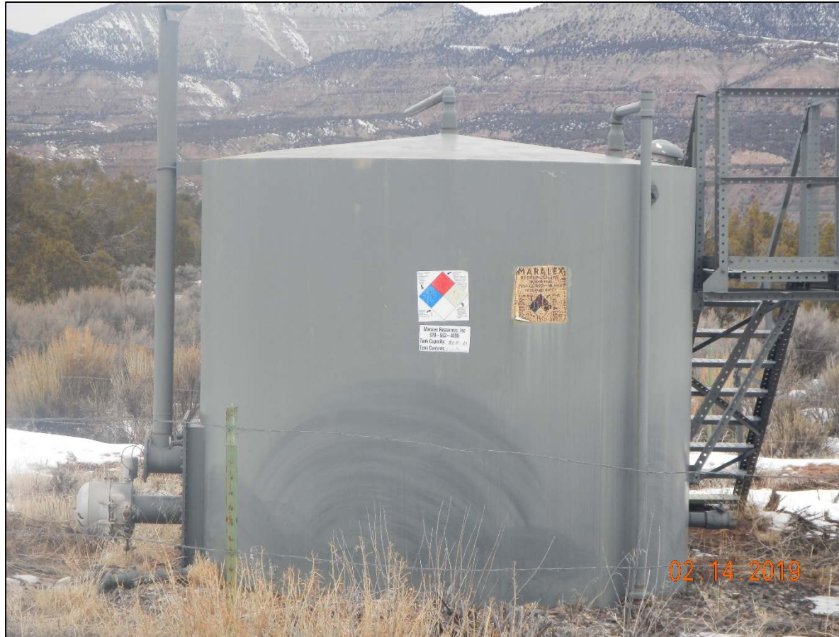
Tank Photo . (labels warn faded, Rubbish inside of berm. )
