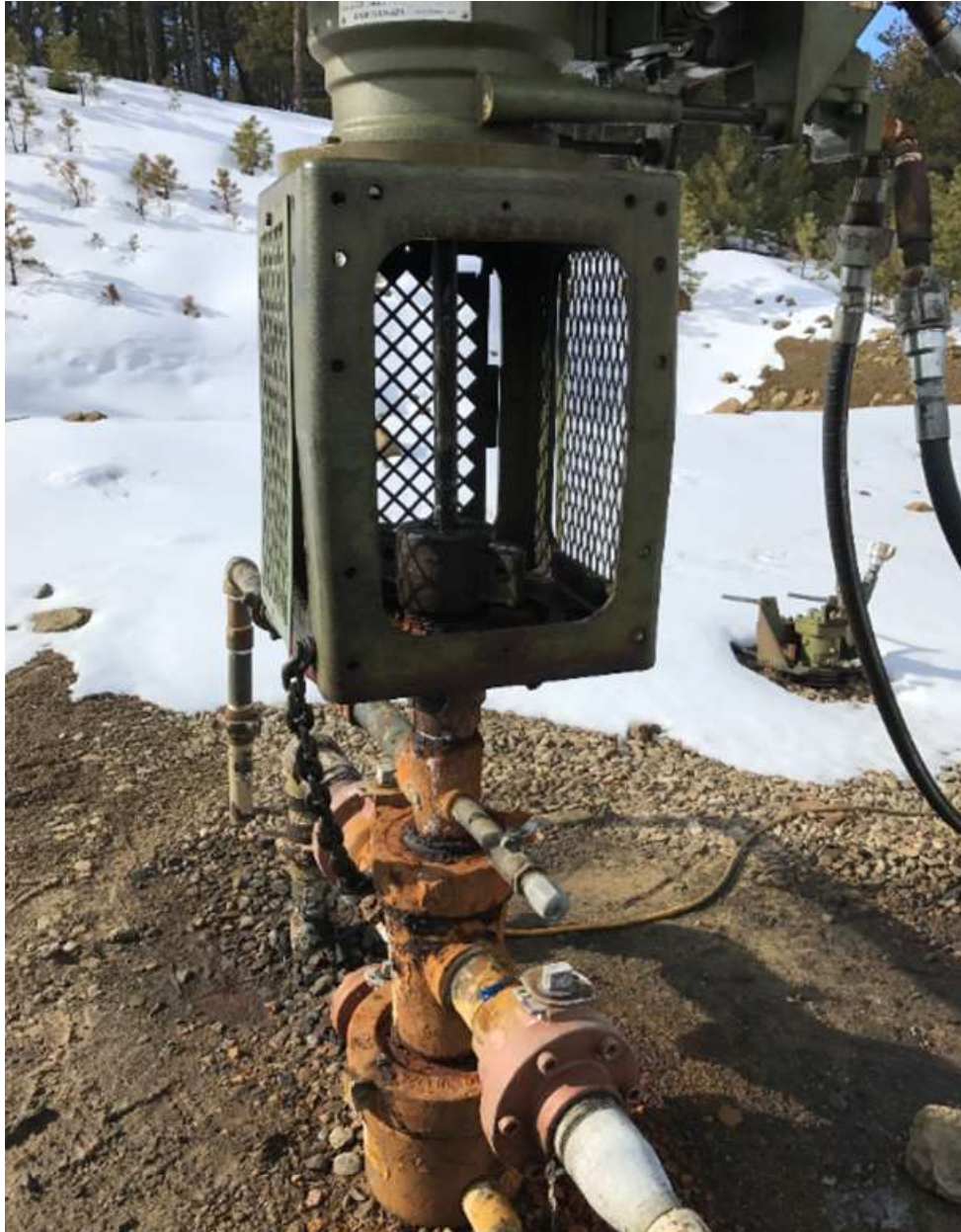
PHOTO 1: THE PACKINGS WERE RELACED, ELIMINATING THE WATER LEAK.
