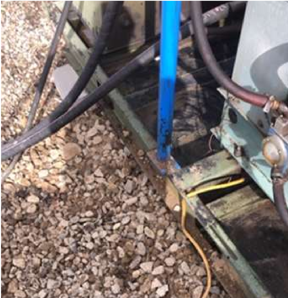
PHOTO 1: THE OIL ACCUMULATION IN THE ENGINE SKID CONTAINMENT AND THE STAINS ON THE GROUND HAVE BEEN CLEANED UP.
