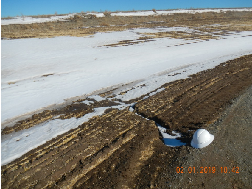
Photo 5. Photo taken from the location, facing Northeast. At the time of this inspection, it appears the Operator has not installed sufficient stormwater and erosion control BMPs in accordance to Rule 1002.f. standards. Photo depicts erosion observed on location.
