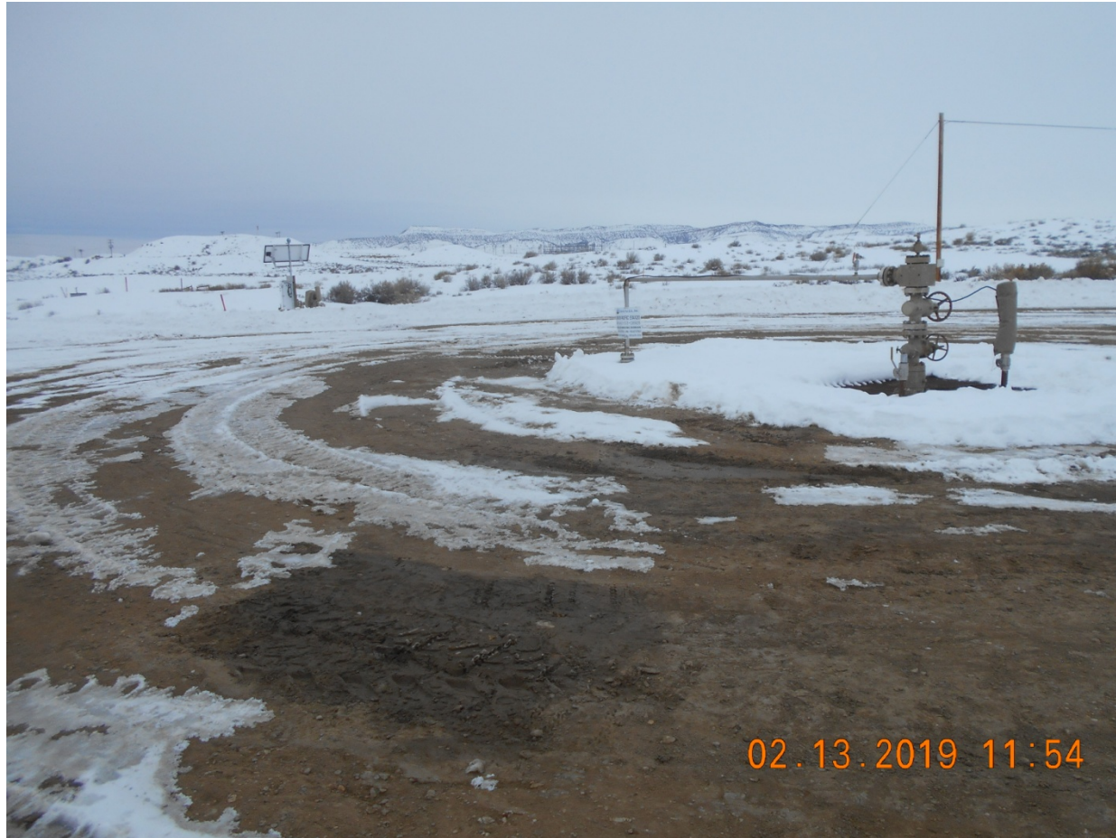
Injection Wellhead
