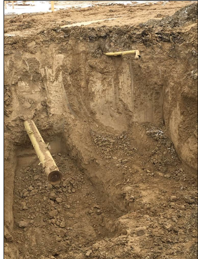
Additional abandoned/unclaimed 2" and 8" pipelines were also capped/removed.
