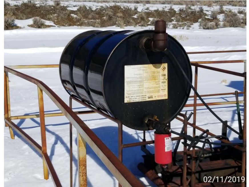
Photo 2. Container without secondary containment.
