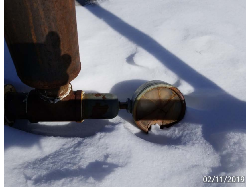
Photo 2. Pressure gauge leaking gas.
