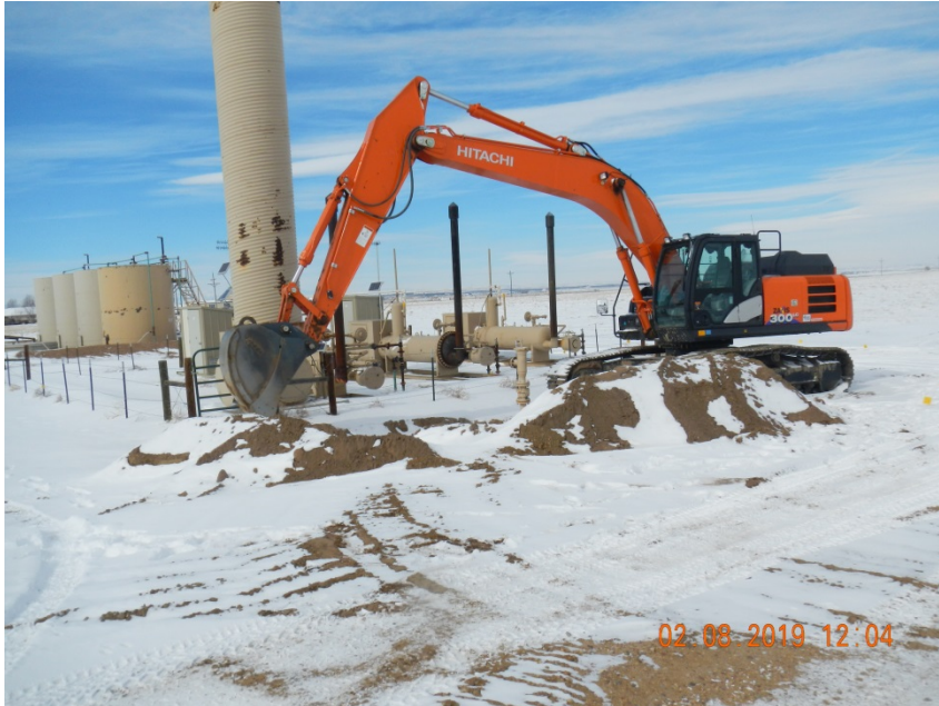
Photo 1. Photo taken from the location, facing Northwest. Appears Operator is in the process of removing the riser at east end of battery location but is still on location.
