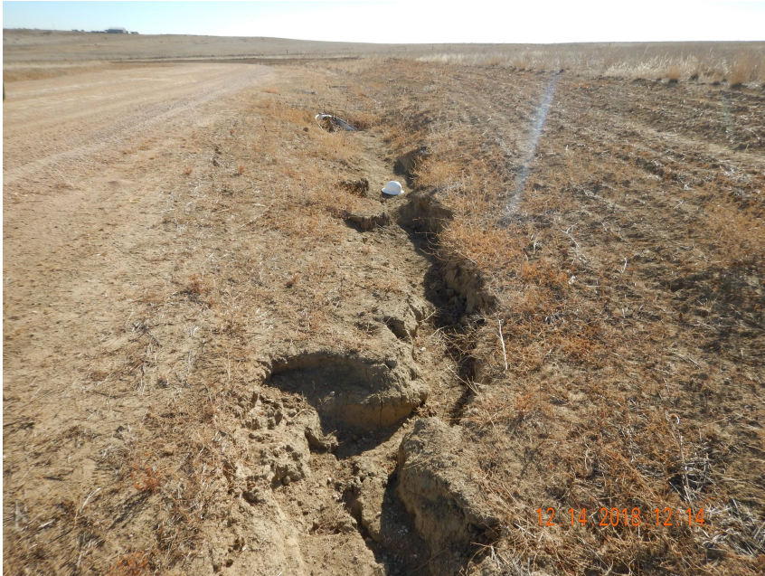
Photo 5. Photo taken along the access road just beyond the entrance of the location on 12/14/2018, facing South. Gully erosion has formed along a section of the access road.
