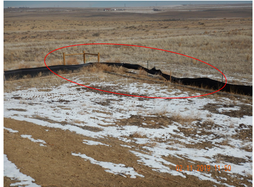
Photo 4. Photo taken from the northeastern location on 2/11/19, facing Northeast. Appears the Operator has made repairs to the silt fence that were previously observed; however, BMP is in need of maintenance.
