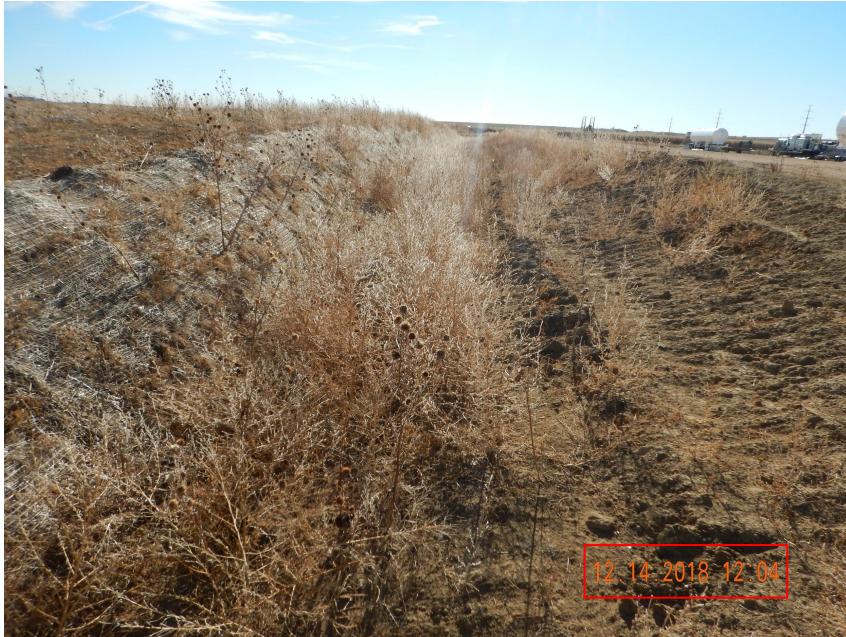
Photo 1. Photo taken from the north eastern topsoil stockpile on 12/14/2018, facing South. Operator has failed to prevent weed establishment on the topsoil stockpile. Note: Appears the Operator attempted to seed the topsoil with desirable vegetation (e.g., blue grama) but weedy, annual vegetation (Kochia) was observed throughout most of the stockpile.
