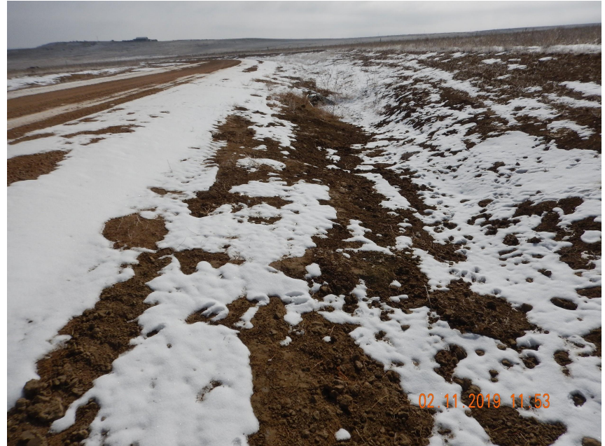
Photo 6. Photo taken along the access road just beyond the entrance of the location on 2/11/19, facing South. Operator has made repairs but has failed to install additional BMPs. It is not sufficient to only make repairs.
