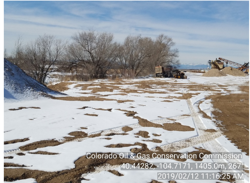
Photo #2 Bucklin 9-36 Battery site Abandoned
