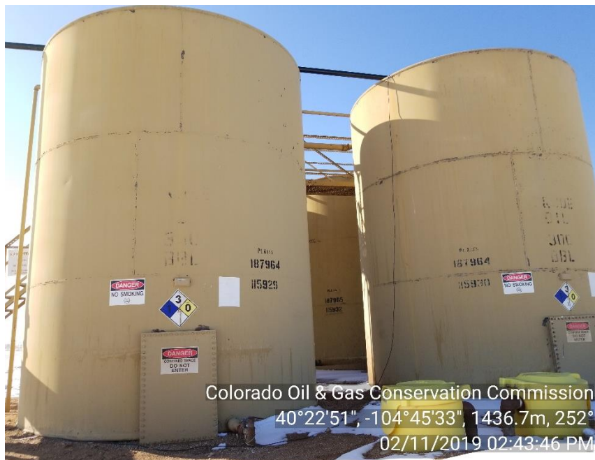
Photo 5: Labeling of tank contents and capacity not visible to road.
