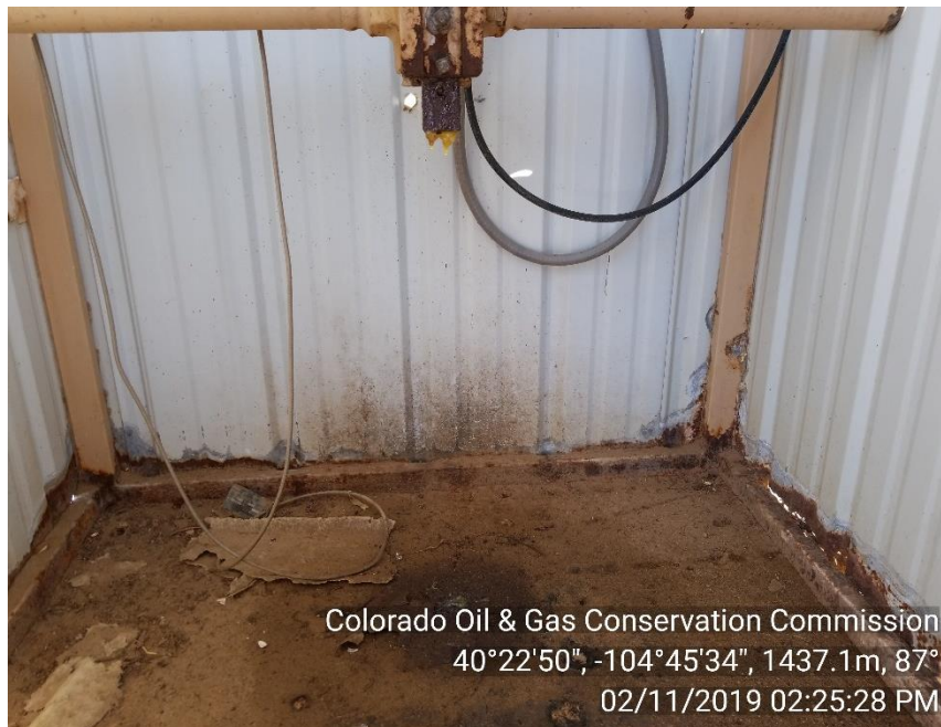
Photo 3: Fluid leaking inside west gas meter house.
