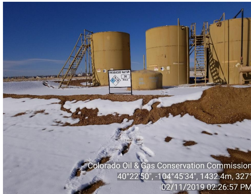
Photo 4: Inadequate berm
