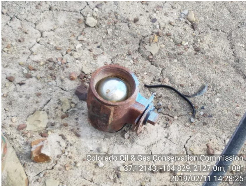
PHOTO 3: UNUSED UNMARKED RISER. NO LO/TO
