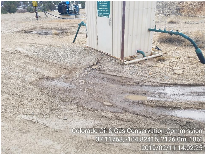
PHOTO 3: APPEARS SEPARATOR IS BEING DRAINED ON LOCATION.
