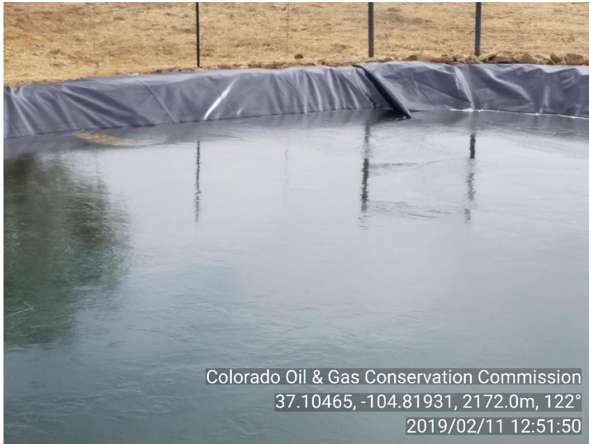
PHOTO 5: PRODUCED WATER APPEARS TO BE ABOVE THE 2' FREEBOARD REQUIREMENT. FREEBOARD MARKER IS NOT INSTALLED ON LOWEST ELEVATION OF PIT.
