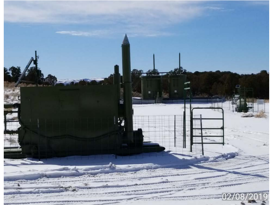
Photo 2. Location looking west.
