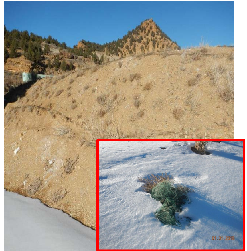
Photo#6: Vegetation establishment on slopes is largely unsuccessful. Insert of netting Debris
