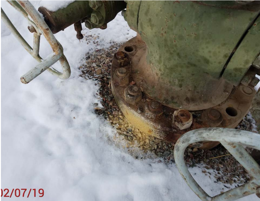
Location Photo #5, stained ground below master valve.
