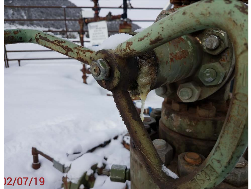
Location Photo #6, Leaking packing on master valve.
