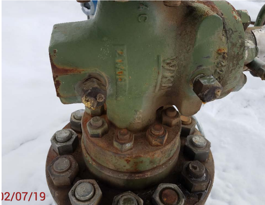
Location Photo #7, Mechanical condition of master valve.
