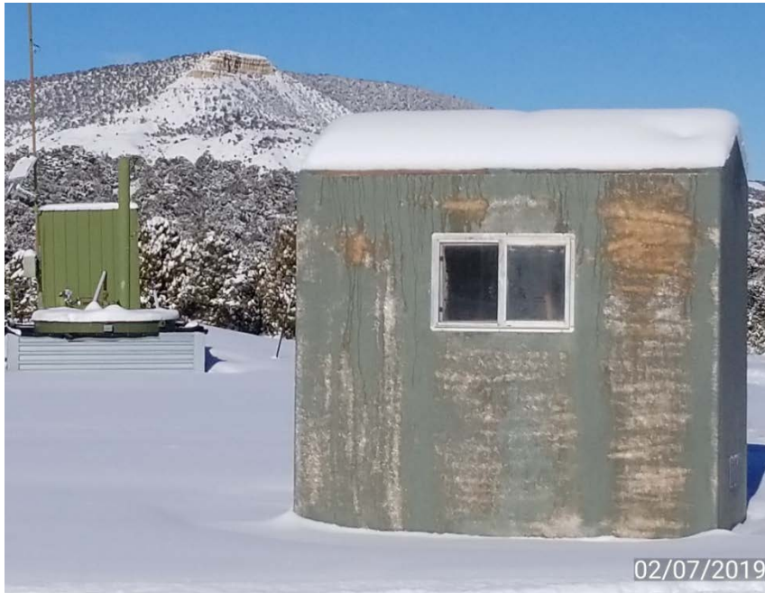
Photo 1. Location looking northwest.
