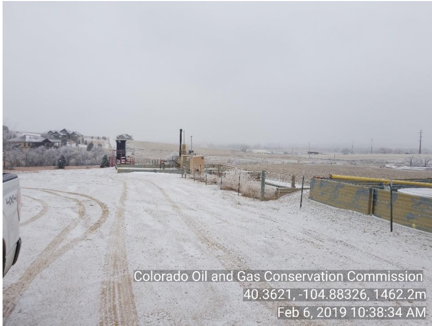
Photo 3 Meter run removed
